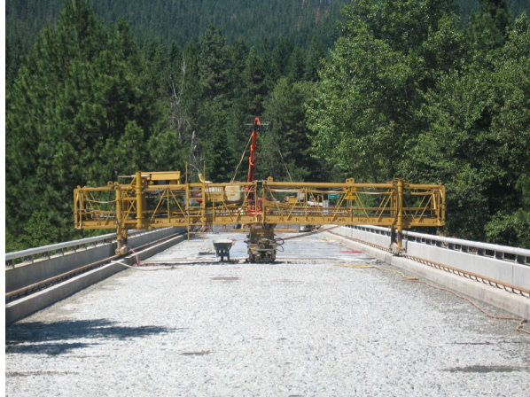
Bidwell Bridge Paver
