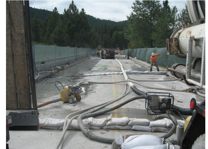
Hoses, pumps, etc. used to supply clean water and collect debris
