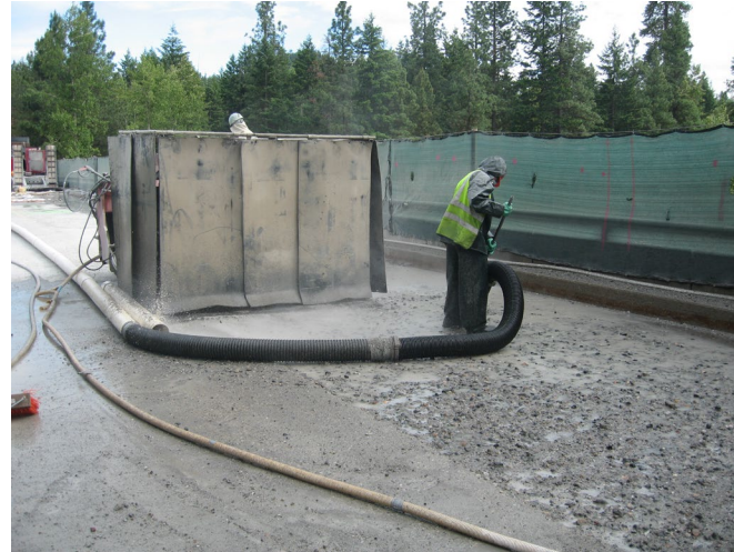
Hydro-Milling with protective screening around water jets
