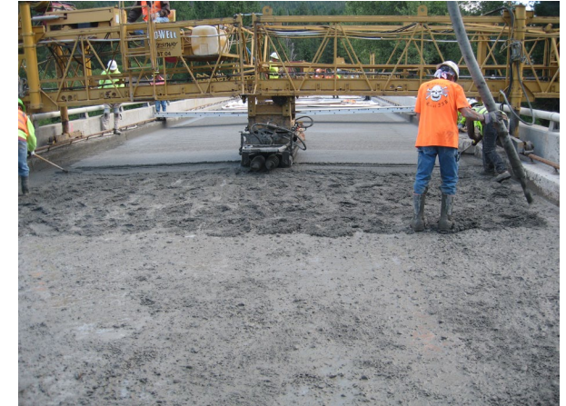
Placing concrete in front of the paver and finishing behind it
