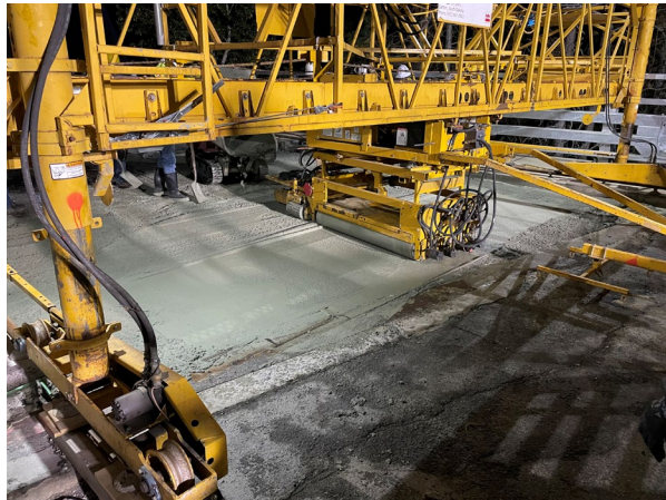
Spreading and leveling concrete with the Paving Carriage
