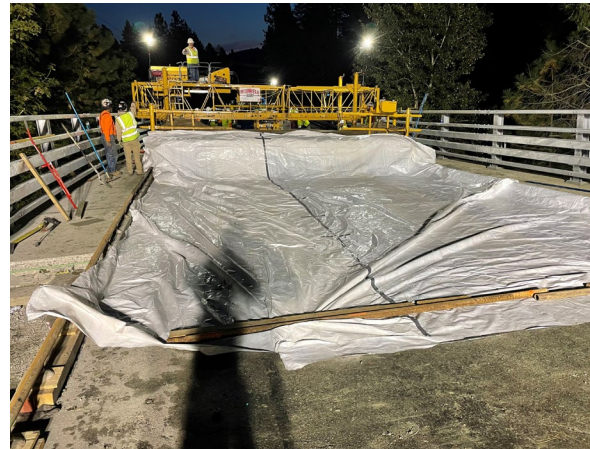
Curing blankets and tarps placed over the finished concrete
