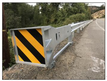
Traffic barriers, such as guardrail, help keep vehicles inside the roadway, away from hazards near the road; they can lessen the severity of crashes. Curve warning signs also alert drivers to take precautions when approaching curves. The photos are from recent road safety improvements made along Squilchuck Road (above) and the Chumstick Highway (right) by Chelan County Public Works.
