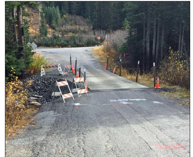
(Right) Temporary repairs to crossing included the installation of two culverts and road repairs.
