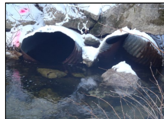
(Above) Washout of culverts from 2015 flood event.
