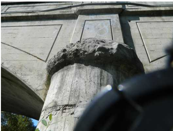
SI-29~I~S~Partially_Repaired_Pier_Cap~2013-10-10_.jpg
