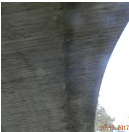
SI-44~G~UP~Typical_Leaching_along_Construction_Joint_in_Arch~2017-10-17_.jpg
