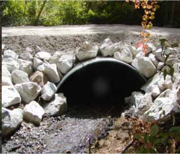
Clear Creek Culvert #1 After Construction in 2007
