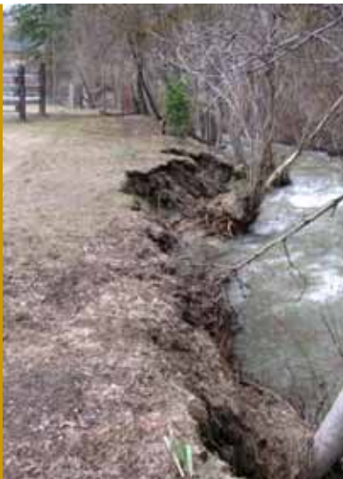
Crowell Riparian (Mission Creek) Before Construction
