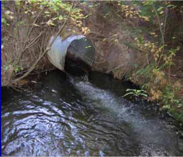
Clear Creek Culvert #1 Before Construction
