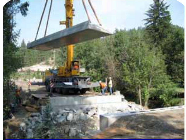
Placement of the bridge deck at the Dolozycki project site.
