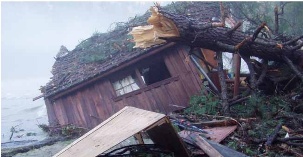
Photo 7 – Destruction of private cabin and damage to upper Company Creek Road during the 2003 flood.
