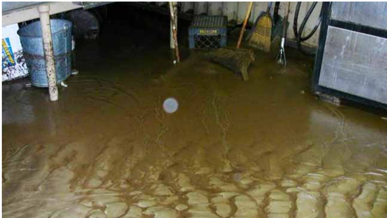
Photo 4 – Floor of NPS Maintenance Shop after 2003 flood.
