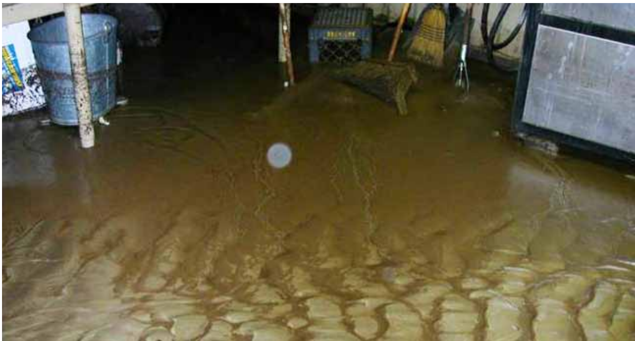
Photo 4 – Floor of NPS Maintenance Shop after 2003 flood.
