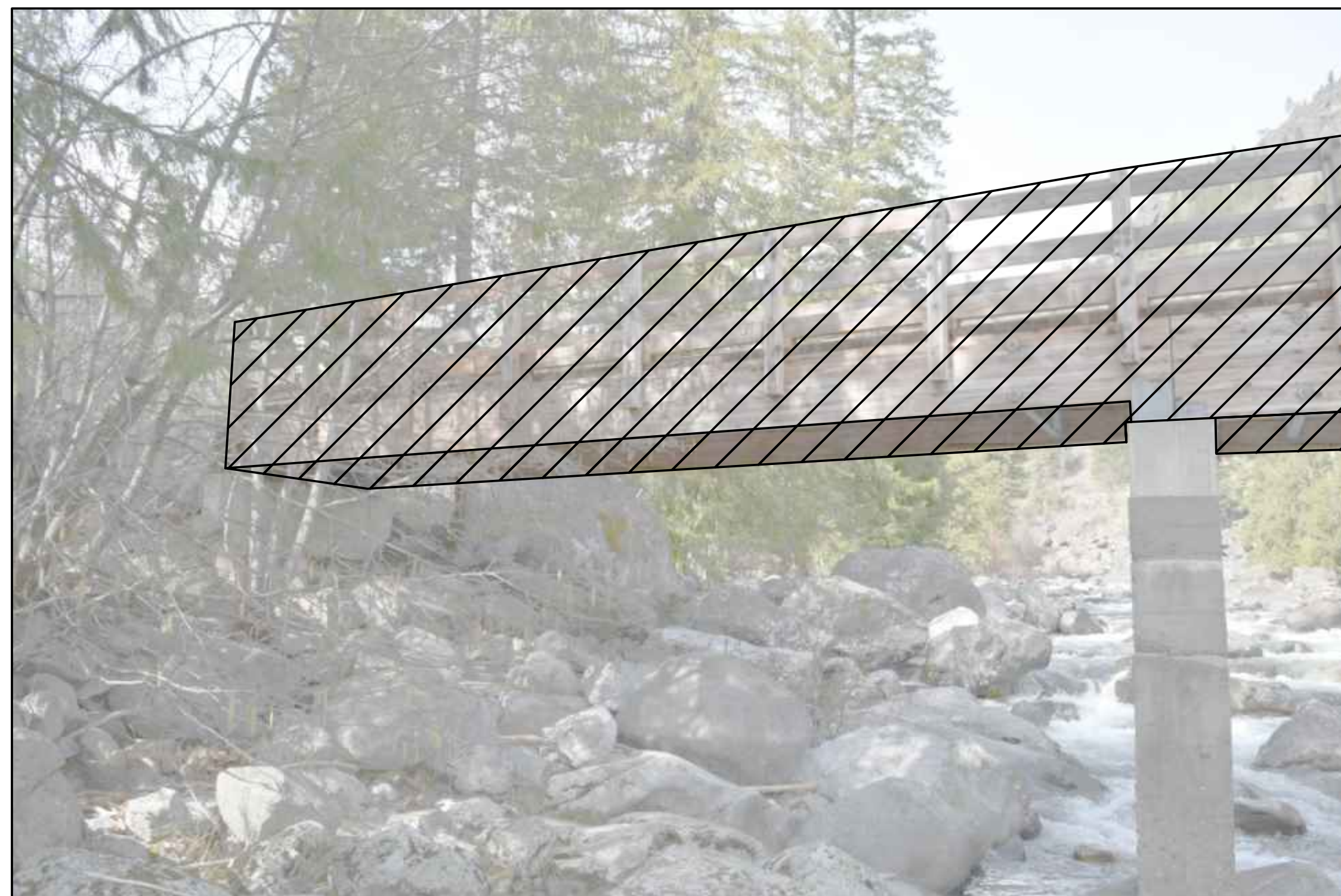
SUPERSTRUCTURE DEMOLITION PHOTO #3 EXIST BRIDGE FOREST SIDE END SPAN SCALE: NTS
