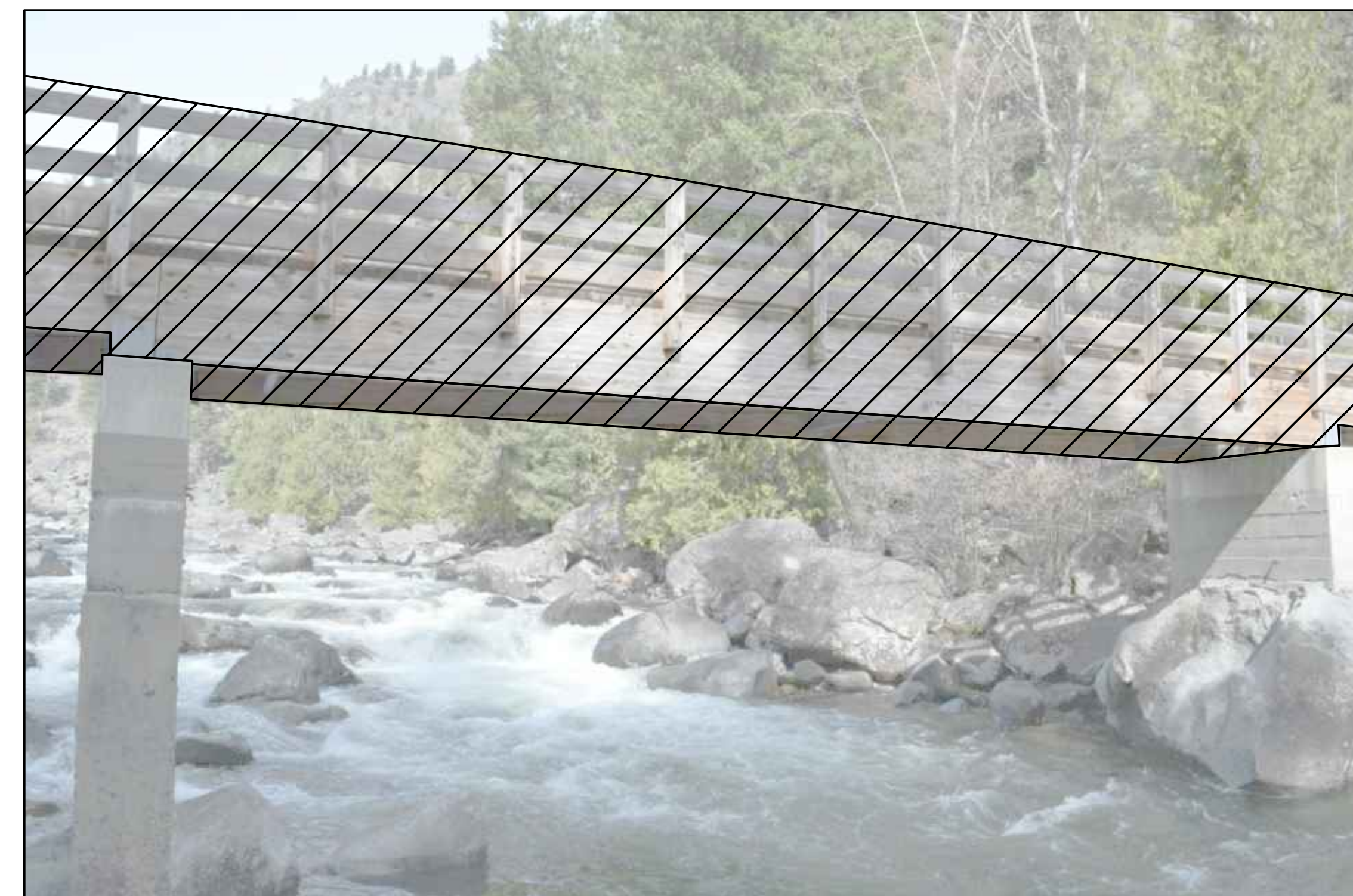
SUPER STRUCTURE DEMOLITION PHOTO #4 EXIST BRIDGE CENTER SPAN SCALE: NTS
