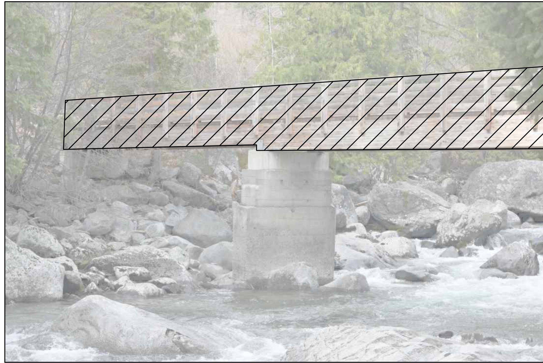
SUPERSTRUCTURE DEMOLITION PHOTO #1 EXIST BRIDGE SCALE: NTS
