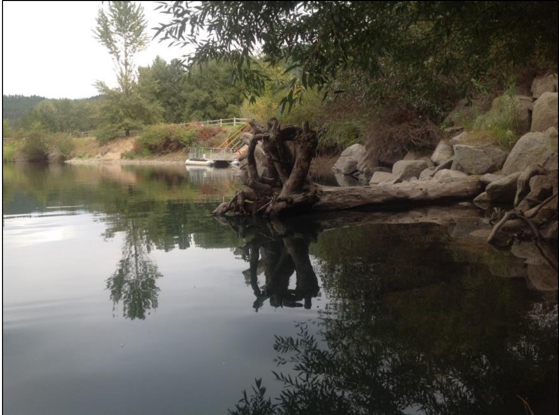
Figure 17. View downstream of single piece of wood with a diameter of 15” and a length of 24’ cabled to rip rap along right bank at RM 2.27.
