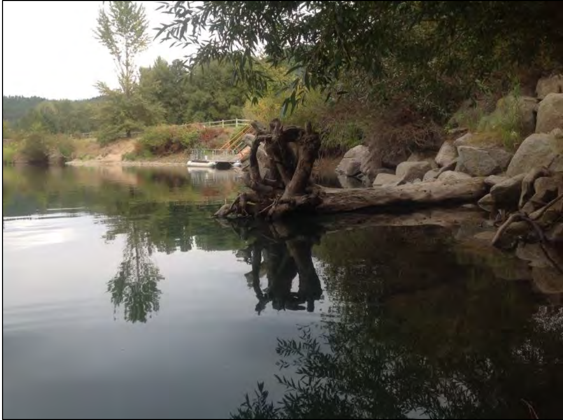
Figure 10. View downstream of single piece of wood with a diameter of 15” and a length of 24’ cabled to rip rap along right bank at RM 2.27.
