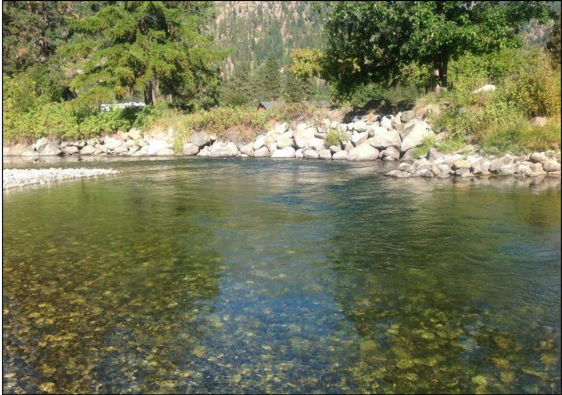
Figure 21. Photo with an example of typical streambank protection using riprap to armor the erodible bank materials.
