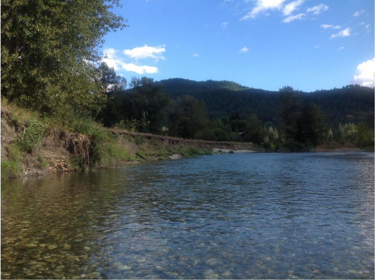
Figure 8. Photo looking upstream along the left bank upstream of the Wenatchee River confluence. The upper bank is composed of fine sediment accumulated in the early 1900s when the Wenatchee River was dammed near Leavenworth. The bank is approximately 12-14 feet high and is just barely overtopped at a 10-year recurrence interval flood.
