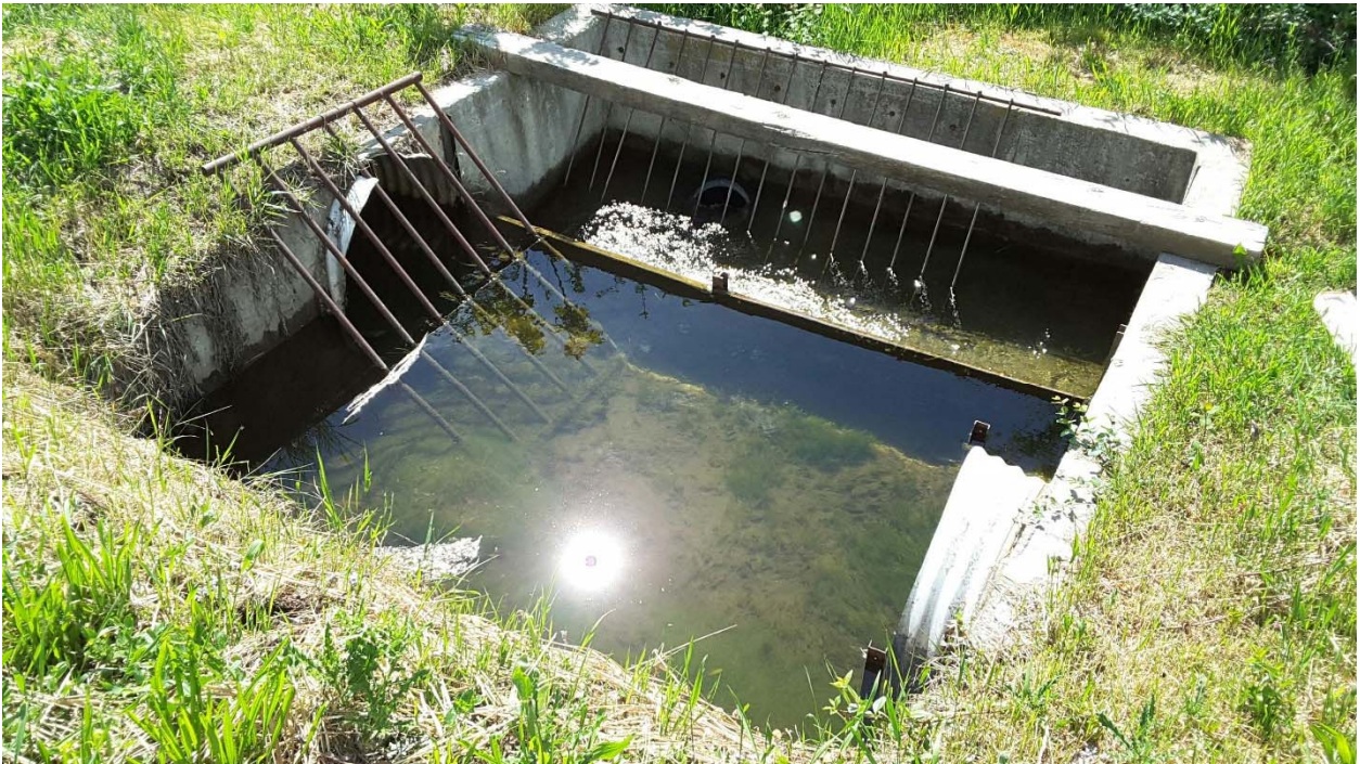
Figure 5-33 IID Division 4 – Control Structure at Williams Canyon Spillway
