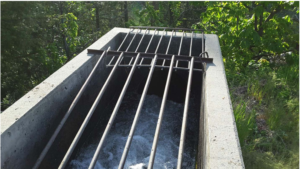
Figure 5-32 IID Division 4 – Derby Canyon Siphon Inlet
