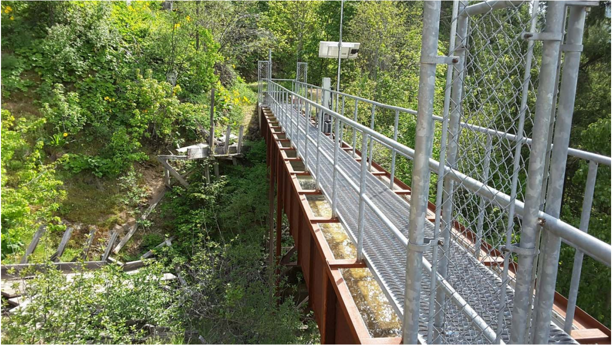
Figure 5-44 PID Canal – Stines Hill Flume and Spillway
