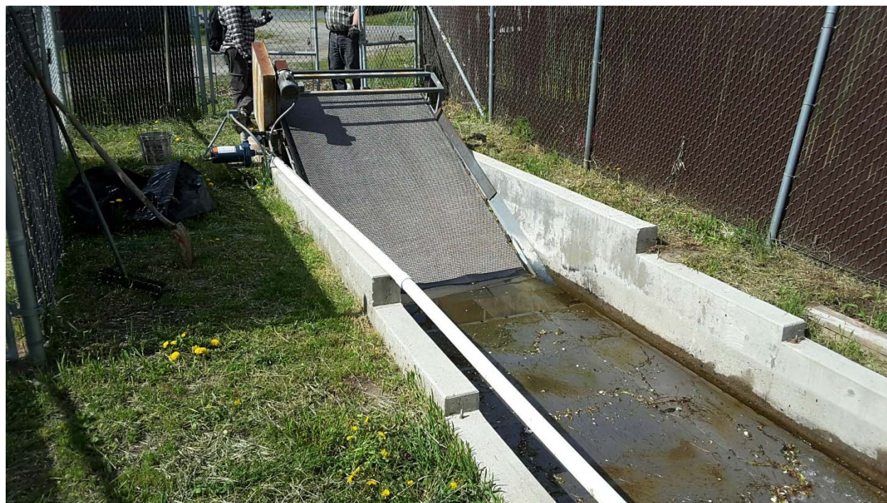
PID Canal – Weed Screen Structure at Inlet to Brender Creek Siphon
