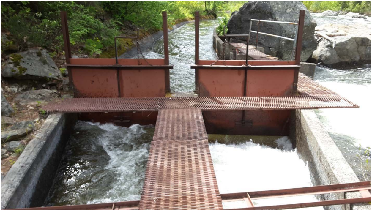
Figure 5-4 IPID Headworks Flume, Head Gates, and Spillway
