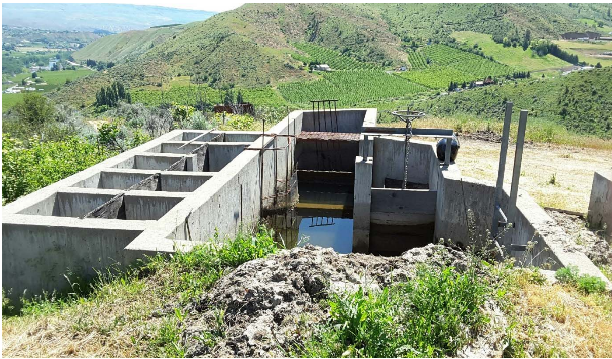
Figure 5-27 Division 3B – Fairview Canyon Siphon Inlet and Spillway
