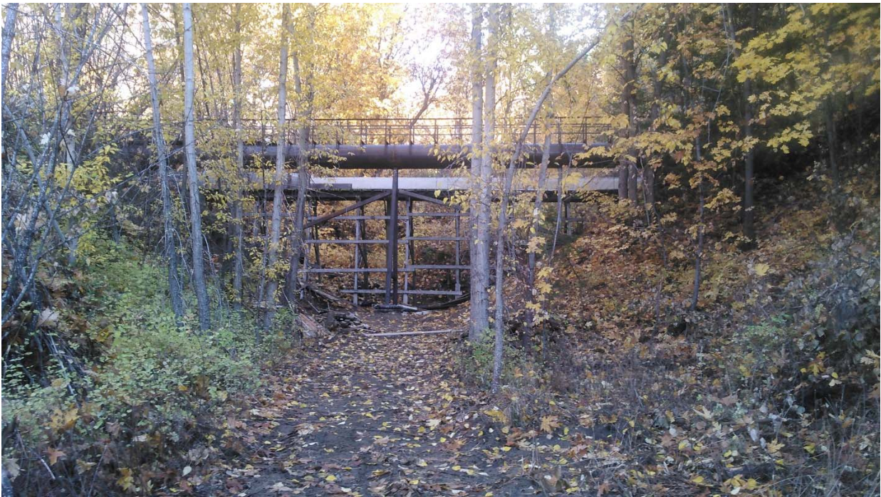
Figure 5-30 IID Division 4 – New Steel Pipe Flume
