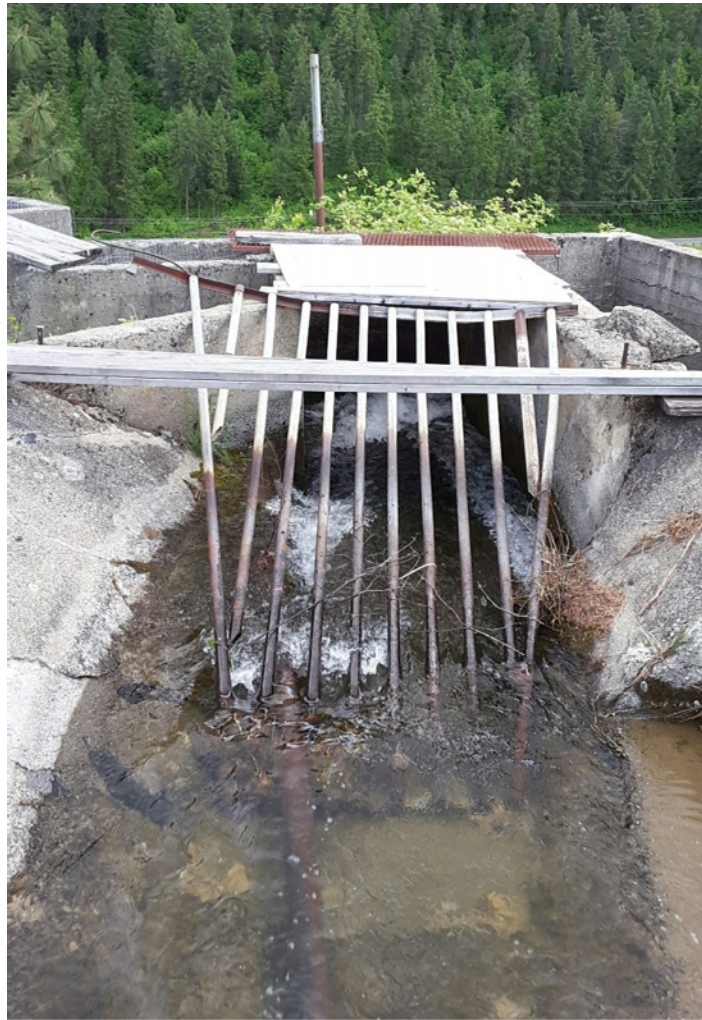
Figure 5-20 Division 3A – Brender Siphon Inlet
