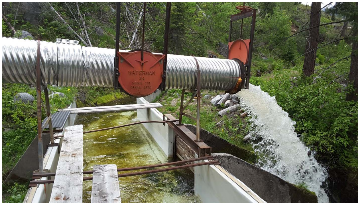
Figure 5-11 Division 1 – Mountain Home Spill
