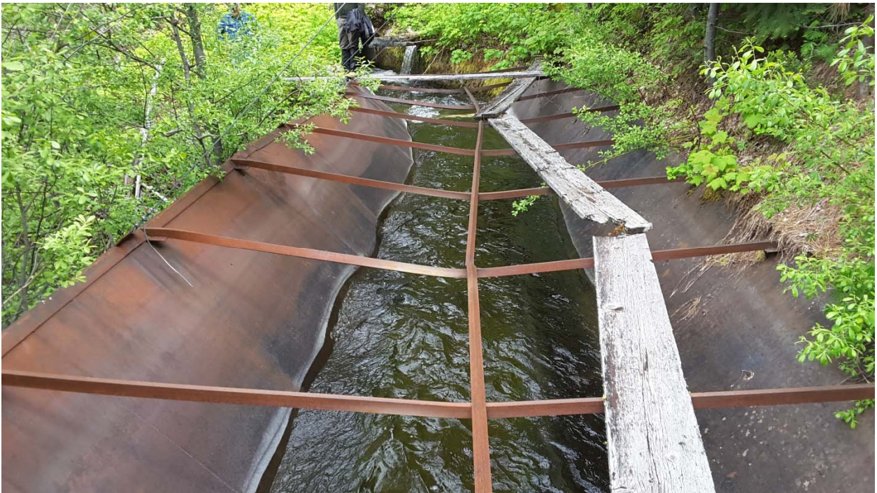
Figure 5-9 Division 1 – Steel Flume
