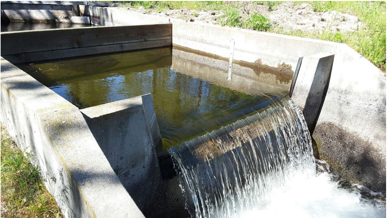
Figure 5-29 IID Division 4 – Posey Weir
