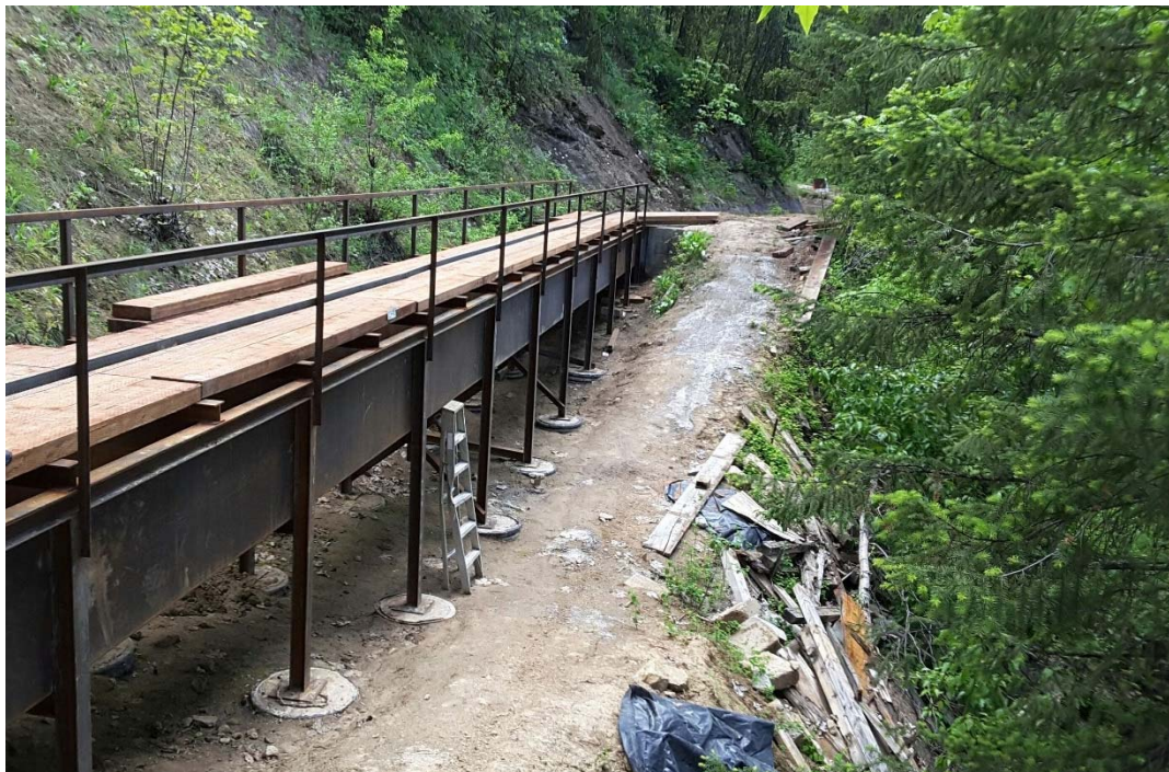
Figure 5-19 Division 3A – Pine Flats Flume
