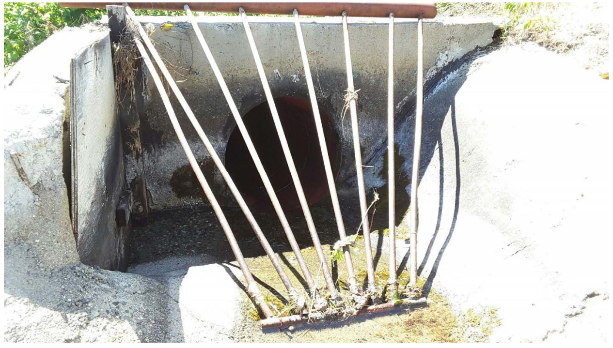
Figure 5-25 Division 3B – Siphon Transition to CMP
