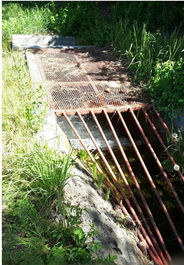
Figure 5-37 IID Division 5 – Chumstick Siphon at Chumstick Creek
