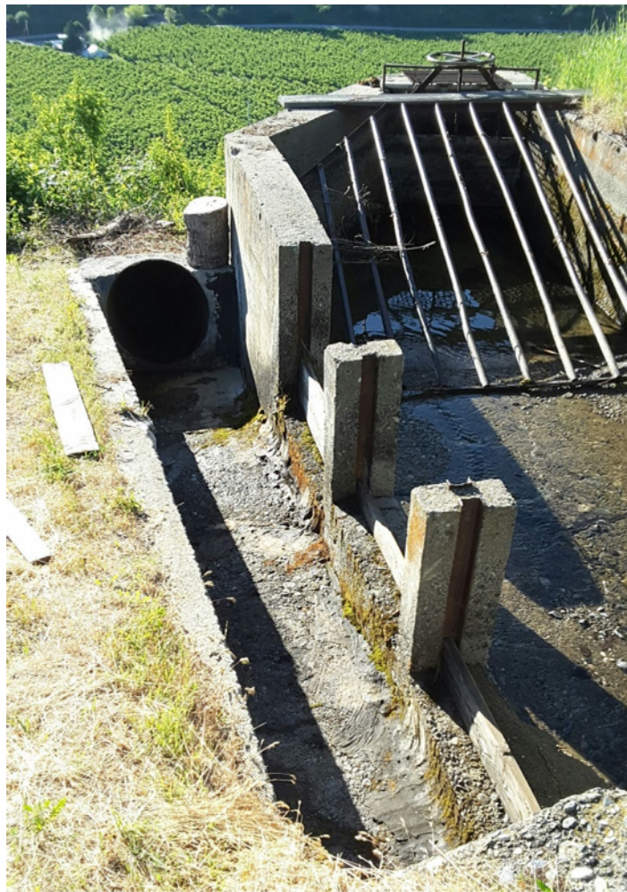
Figure 5-22 Division 3A – Mission Creek Spill and Siphon Inlet
