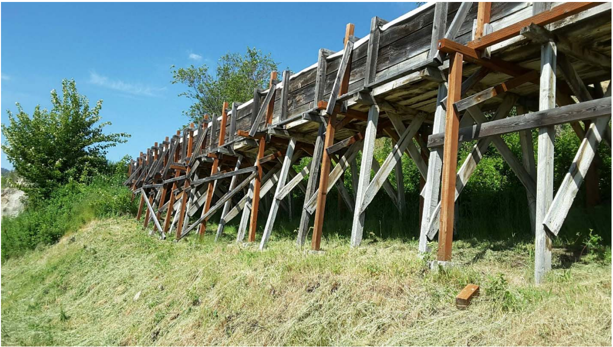
Figure 5-45 PID Canal – Wood Flume
