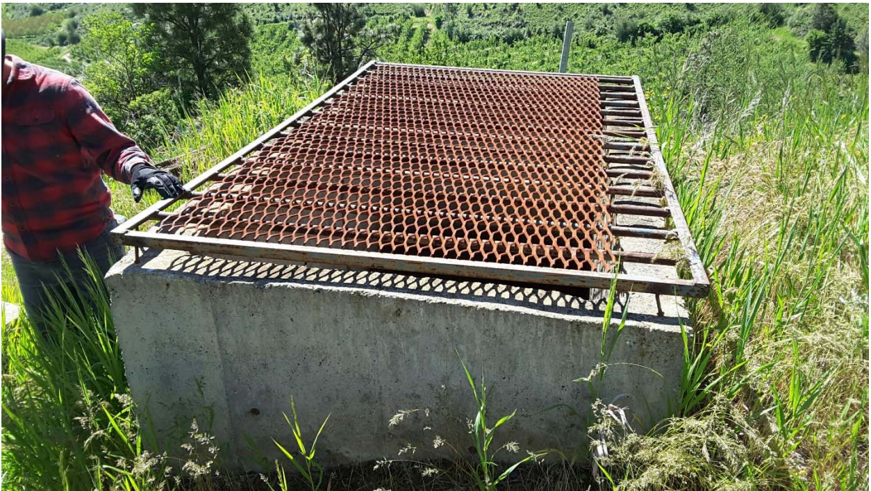
Figure 5-26 Division 3B – Siphon Outlet
