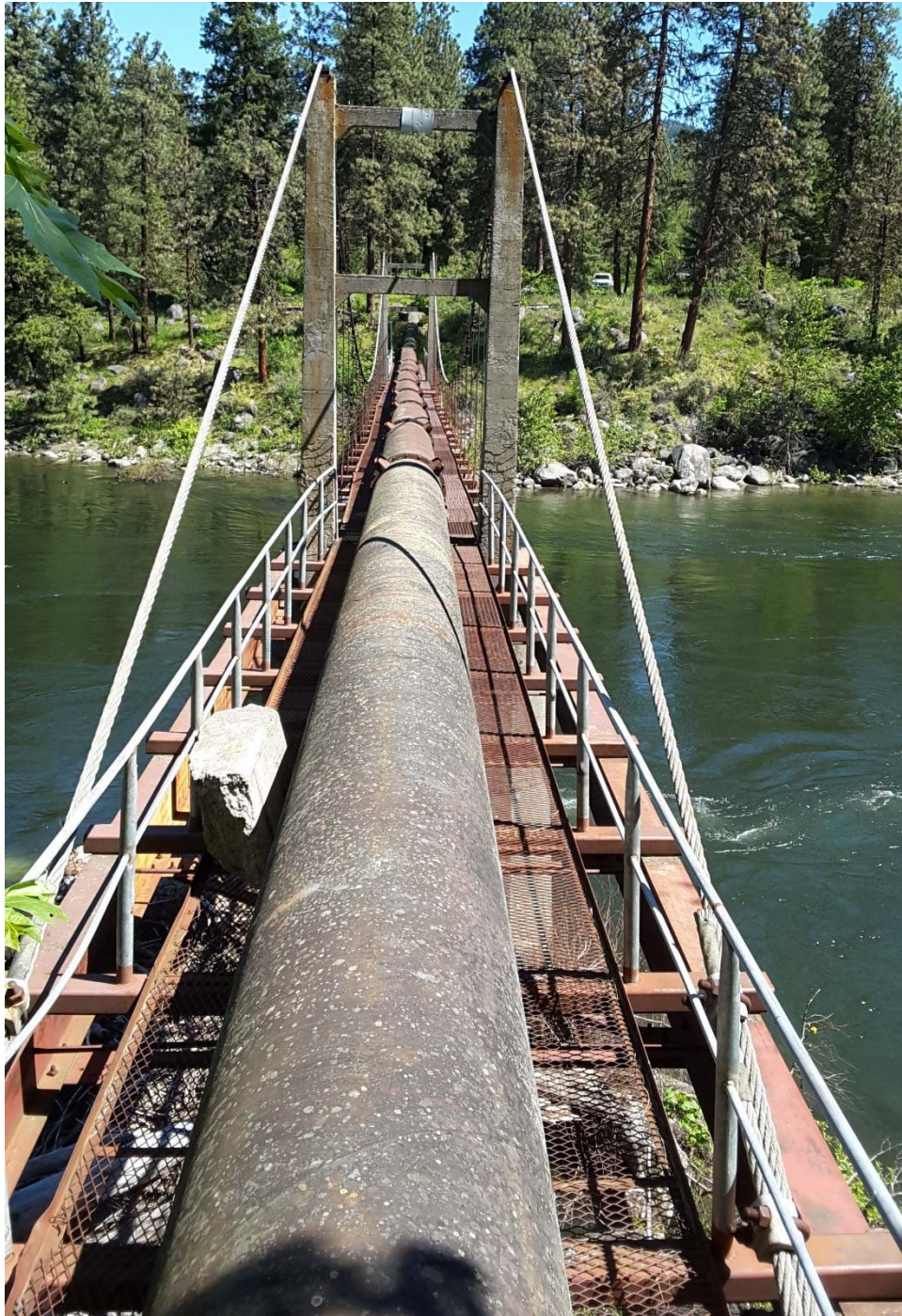
Figure 5-28 Leavenworth Siphon and Pipe Bridge
