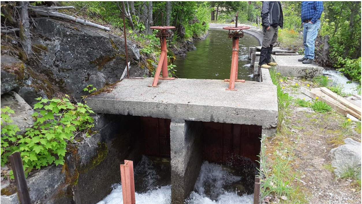
Figure 5-6 Division 1 – Snow Creek Spillway and Gates
