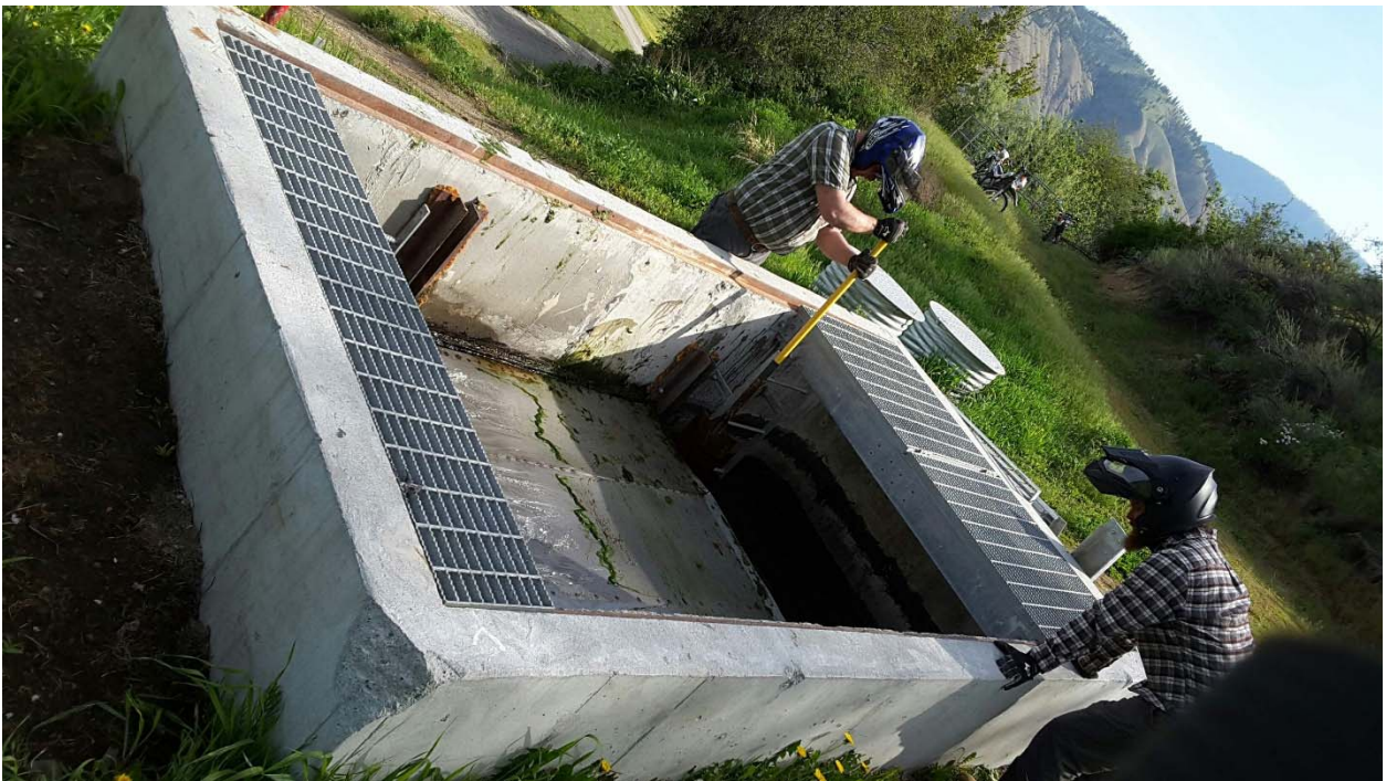
Figure 5-47 PID Canal – Gated Control Box
