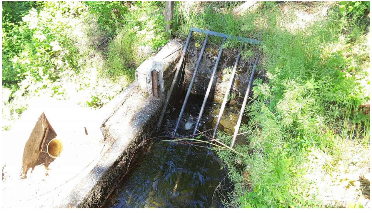
Figure 5-35 IID Division 5 – Moe Siphon Inlet and Spill
