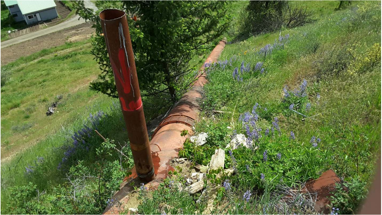
Figure 5-18 Division 3A – Maxwell Siphon Inlet
