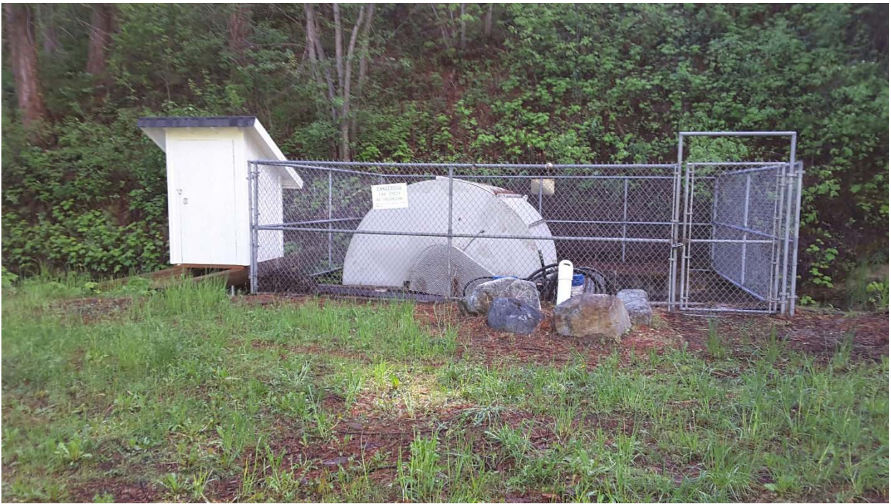
Figure 5-41 PID Canal – Fish Screens
