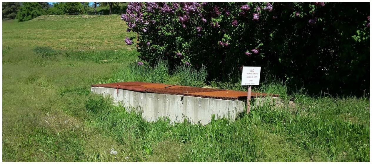
Figure 5-36 IID Division 5 – Fox Spillway Box
