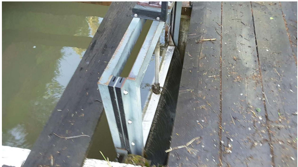
Figure 5-43 PID Canal – Fryburger Spillway Structure
