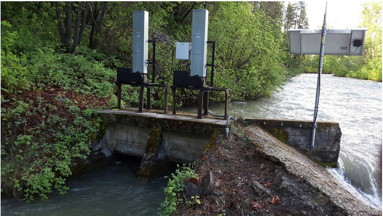
Figure 5-40 PID Canal – Intake Structure and Head Gates
