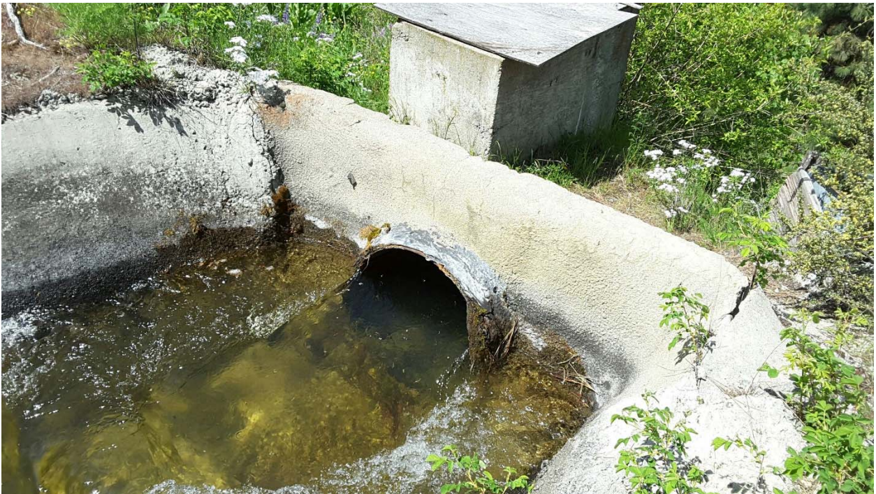
Figure 5-17 Division 3A – Peshastin Siphon Outlet
