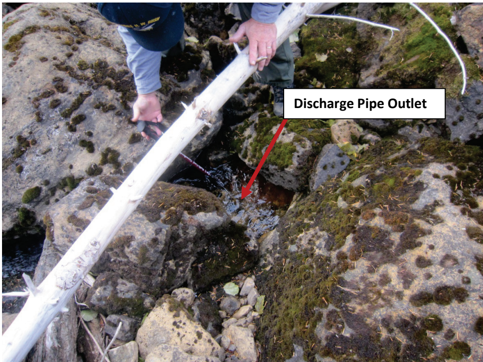
Photograph 10 – Discharge Pipe Outlet to Eightmile Creek
