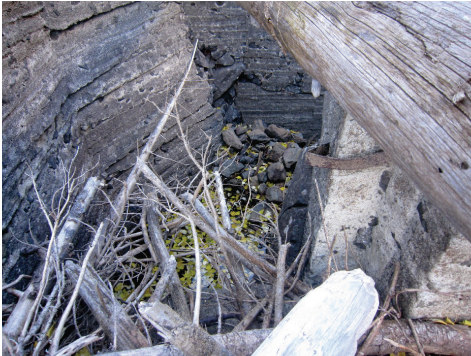
Photograph 5 – Primary Spillway Well
