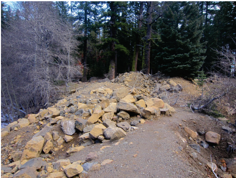
Photograph 2 – Remnants of Earthen Embankment
