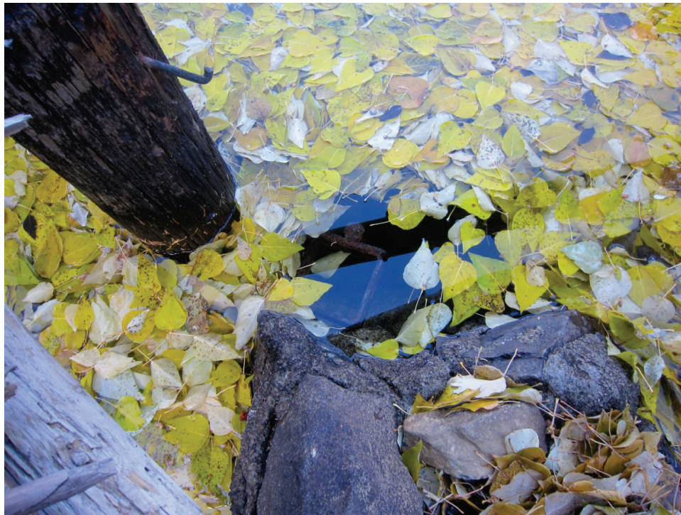
Photograph 7 – Top of Outlet Gate
