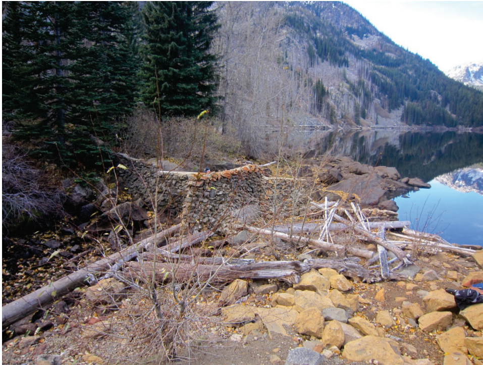
Photograph 1 – Masonry Rock and Concrete Dam from Earthen Embankment
