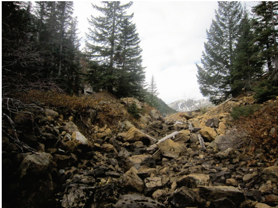
Photograph 11 – Overflow Spillway Channel
