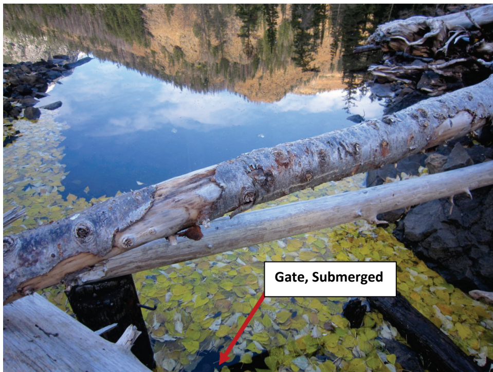
Photograph 8 – Outlet Gate Location
