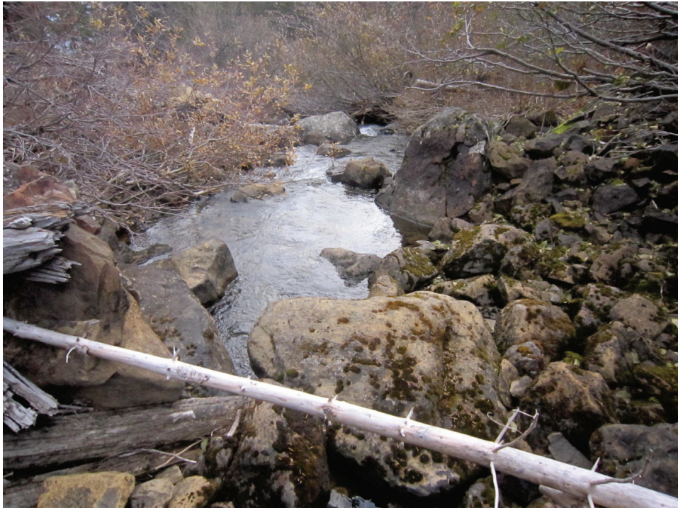
Photograph 9 – Discharge Pipe Outlet to Eightmile Creek
