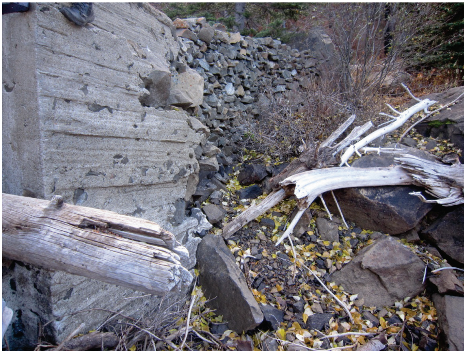
Photograph 6 – South Leg of Masonry Rock and Concrete Dam
