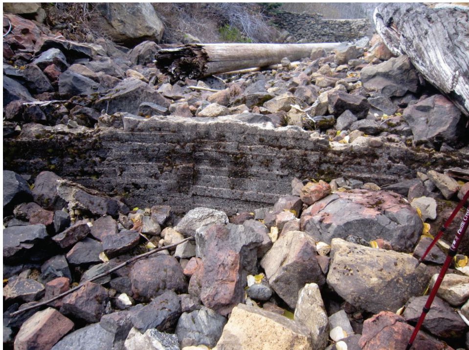
Photograph 12 – Overflow Spillway Channel with Exposed Cutoff Wall
