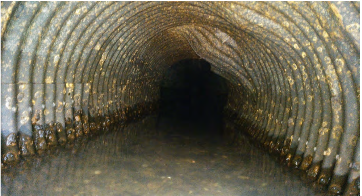
Photograph 11 Low-Level Outlet Pipe, Near Pipe Outlet
