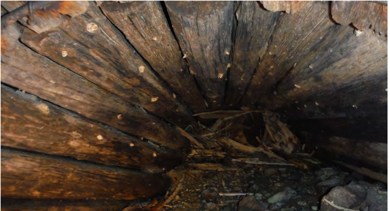
Photograph 9 Low-Level Outlet Pipe, Log-Stave Section
