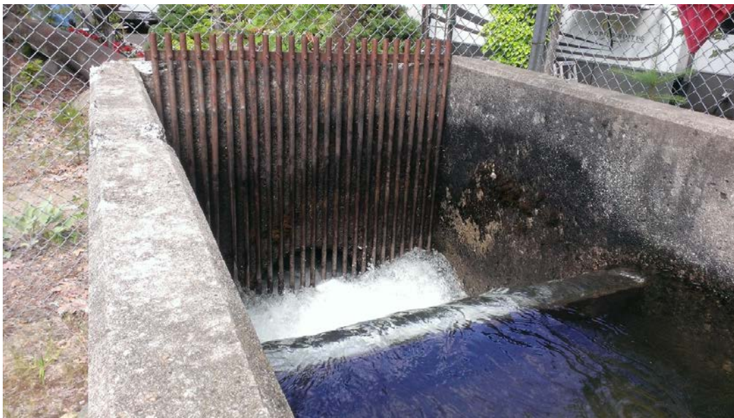
Photograph 8 – Weir, Pipe Inlet, Debris Rack
