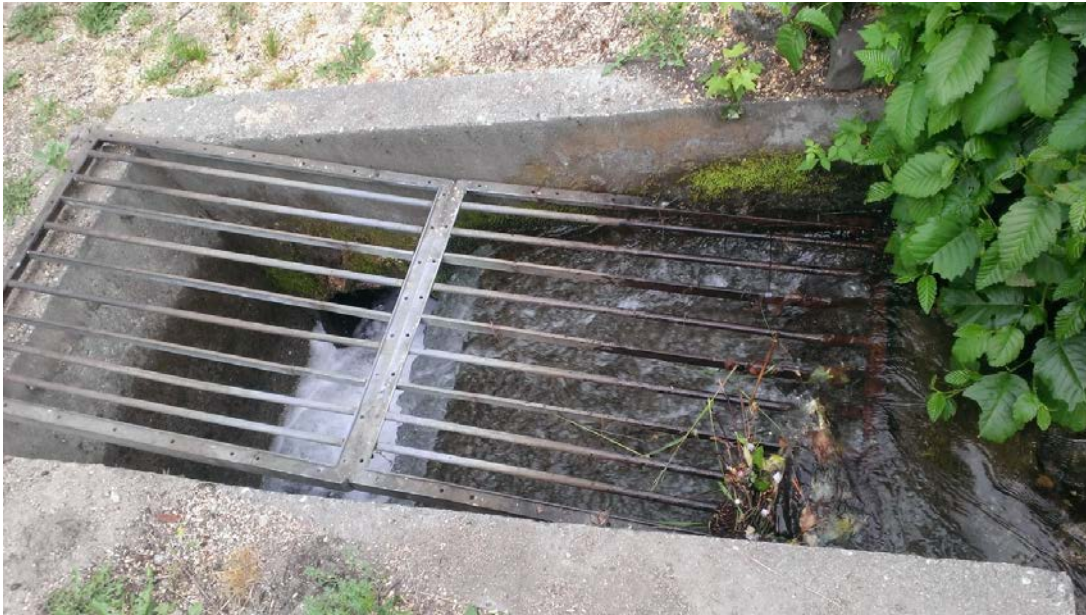
Photograph 19 – Inlet to Tailwater Pipeline at Downstream End of System
