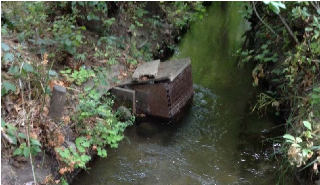
Photograph 17 – Lateral Intake Structure West of Icicle Road
