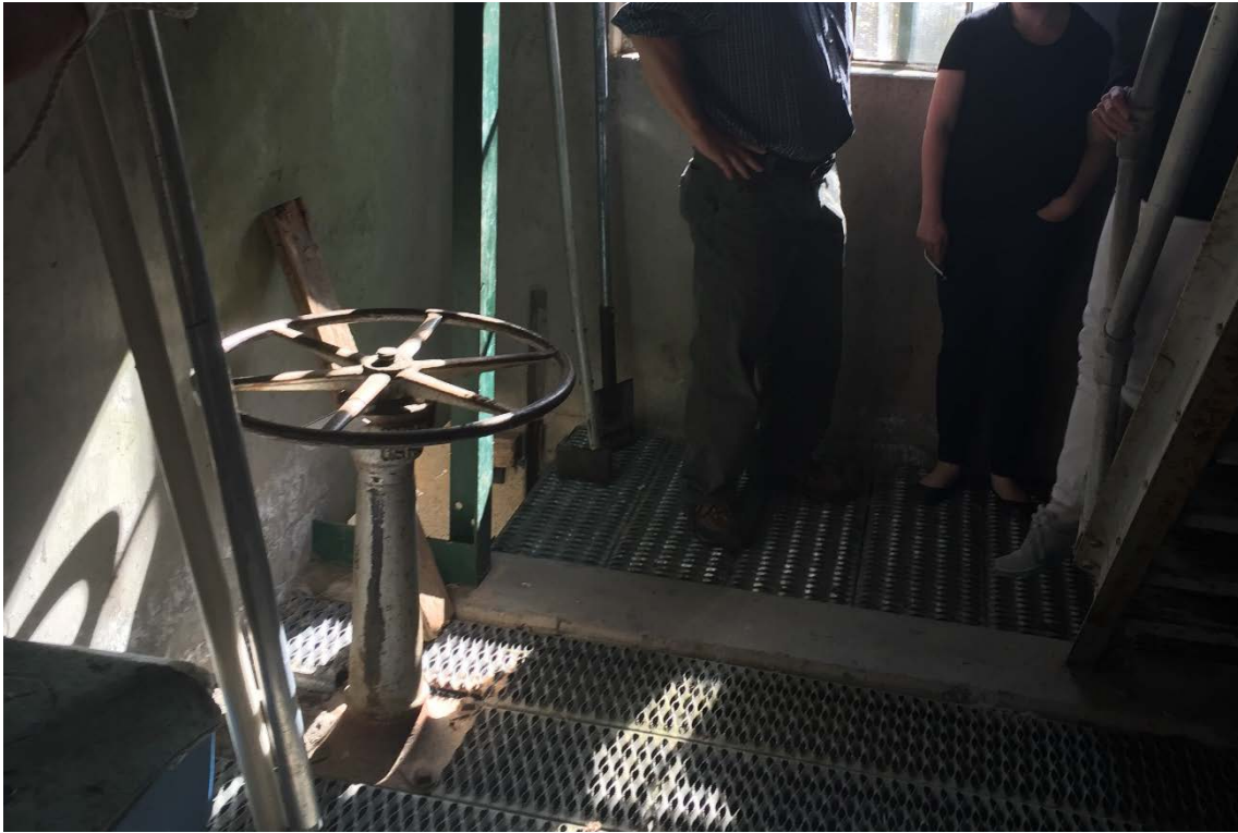
Photograph 3 – Inside Control House with Control Gate Operator
