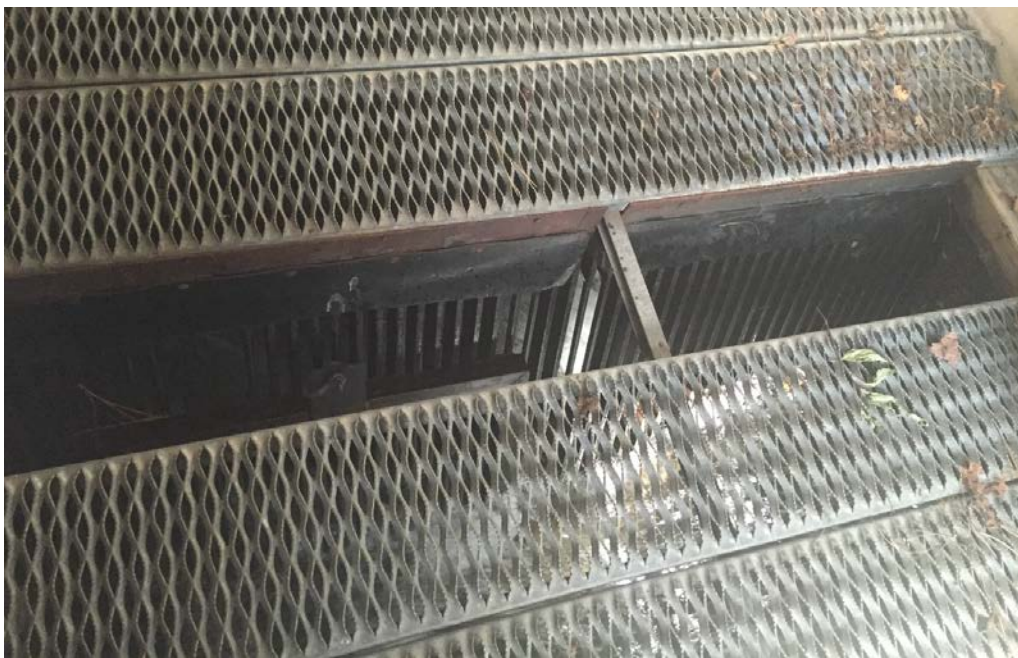
Photograph 2 – Debris Rack at Inlet to Diversion Pipeline under Control House
