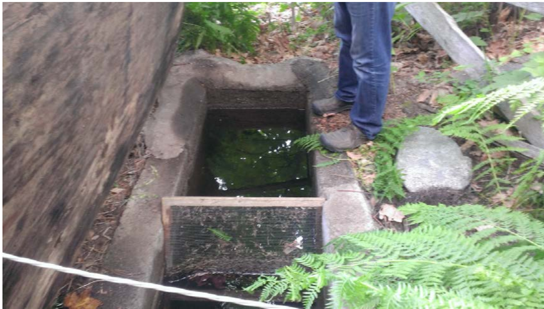
Photograph 18 – Lateral Intake Structure West of Icicle Road
