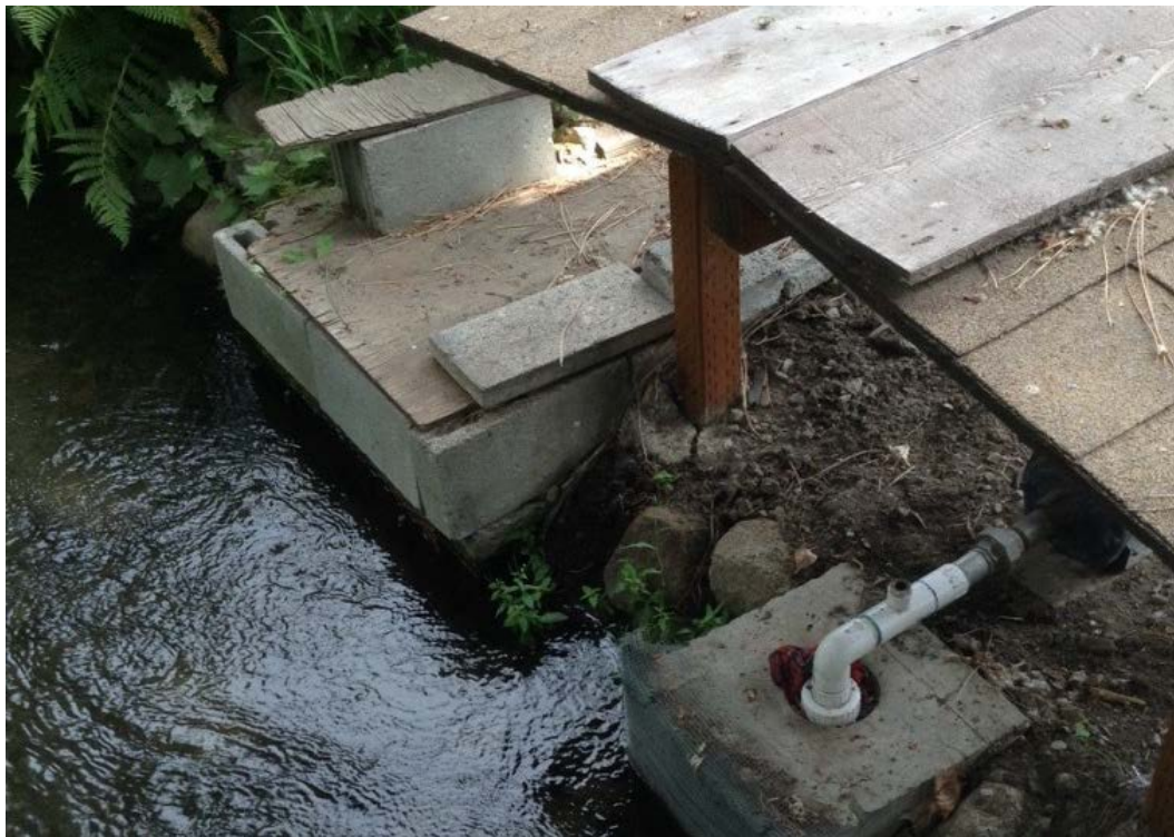
Photograph 16 – Typical Pumped Turnout West of Icicle Road
