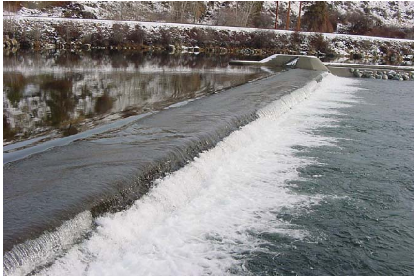
Photograph 5 Dryden Dam, Wenatchee River, with rubber bladder in deflated position.
