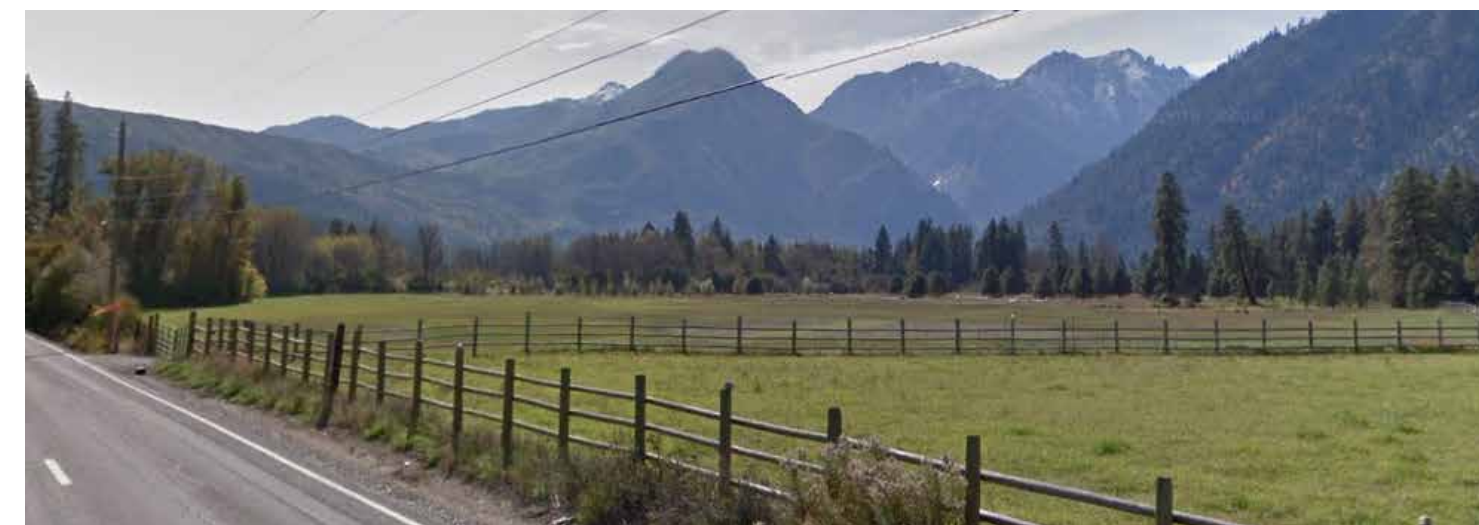
East Leavenworth Road provides a scenic route for recreation enthusiasts, but existing conditions including narrow roadways and bridges create dangerous conditions.
