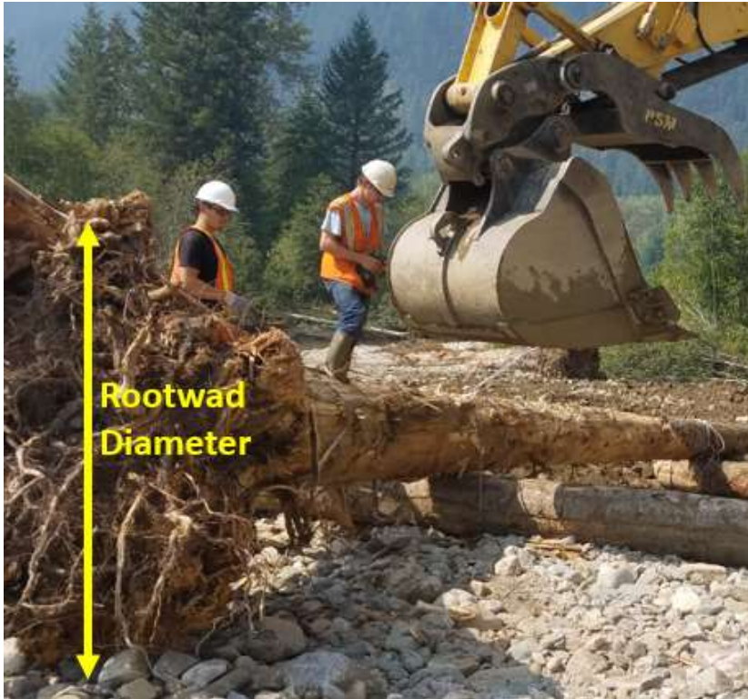
Figure 1. Example of where to measure rootwad diameter.
