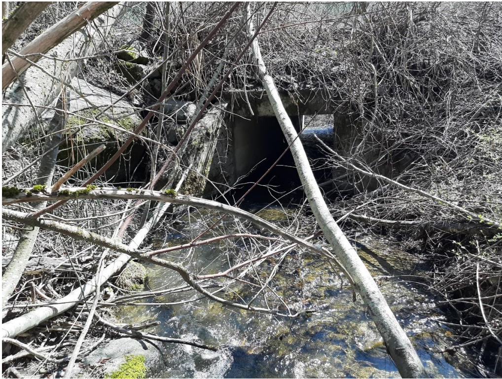
Existing Culvert Upstream looking downstream
