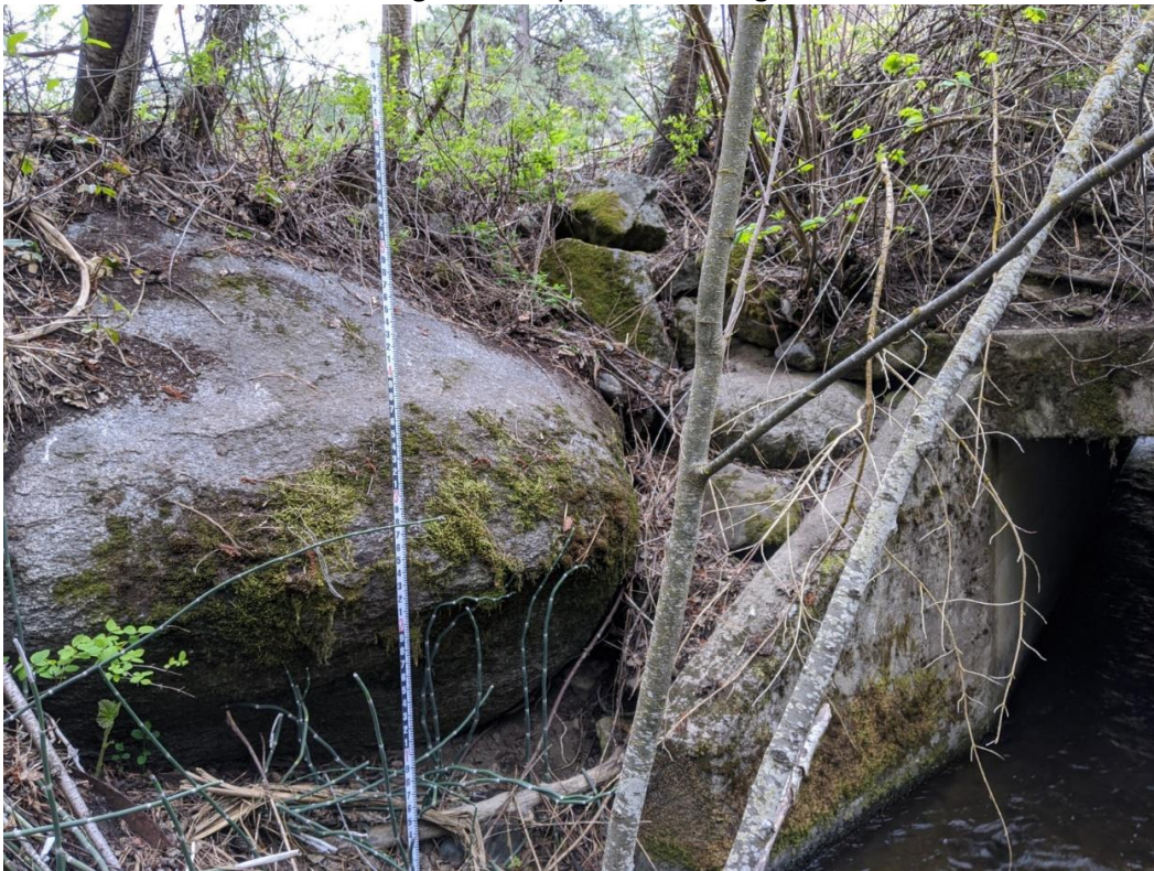
Large Boulder on left bank of culvert
