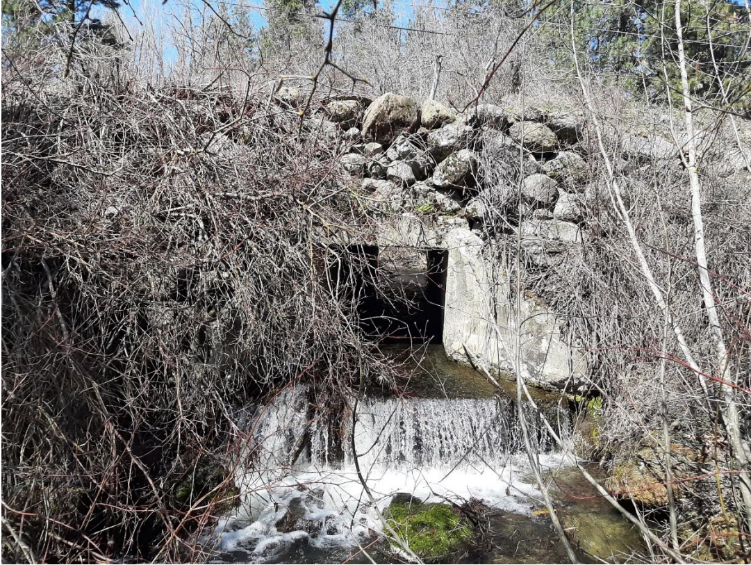
Downstream of existing culvert looking upstream
