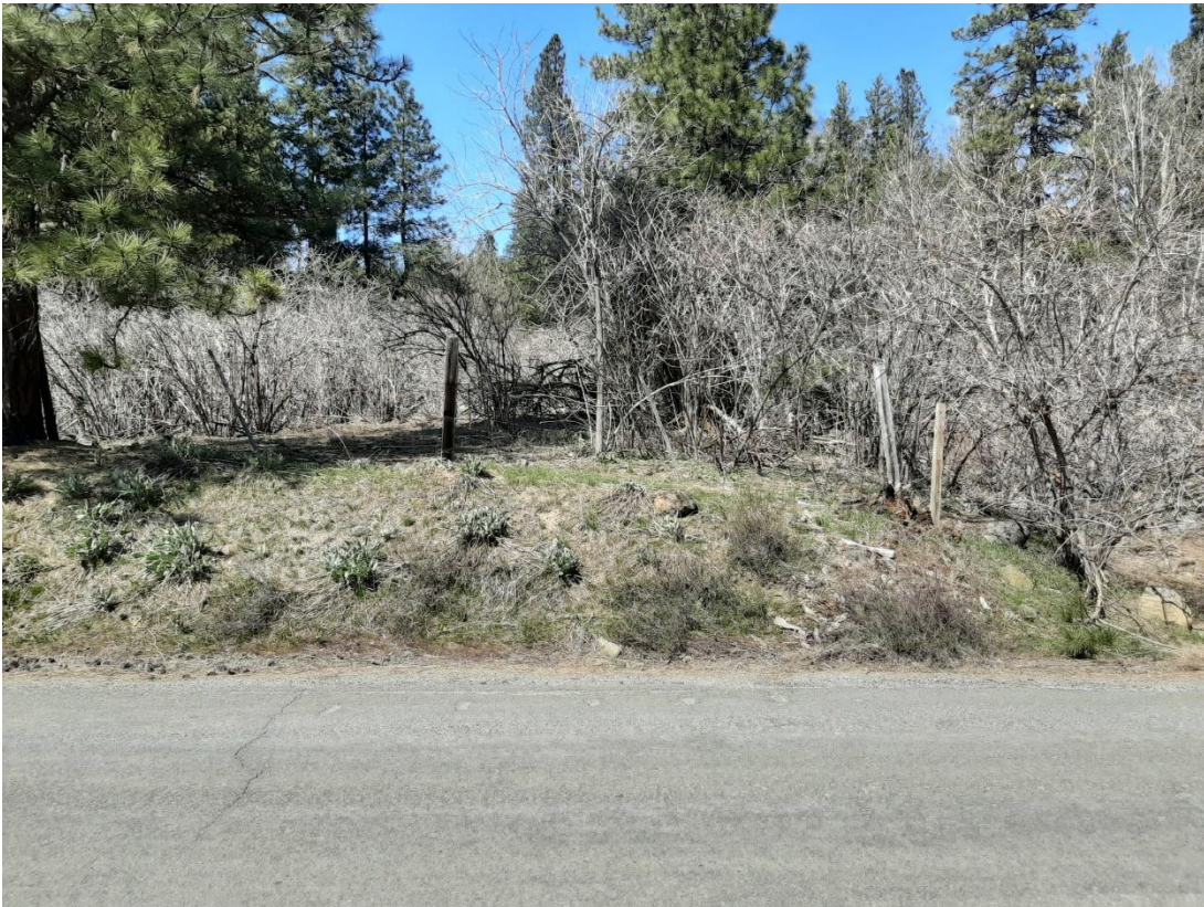
Existing livestock fence (post & barbed wire) to be relocated and replaced
