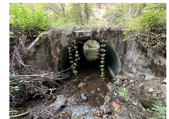
View U/S End Culvert
