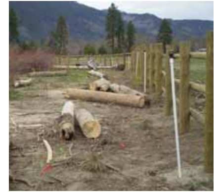
Irrigation and fence project to keep livestock out of riparian area.
