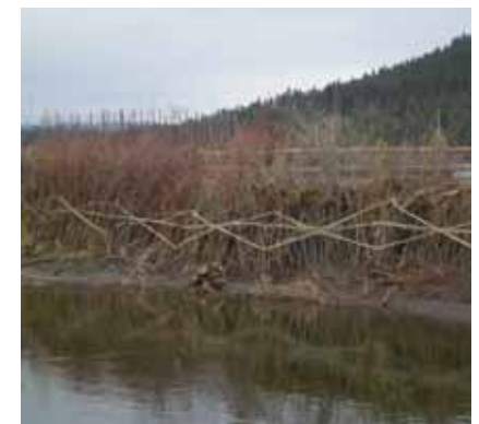
Stream bank stabilization with staking willow cuttings.
