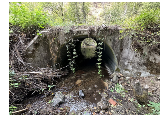
View U/S End Culvert
