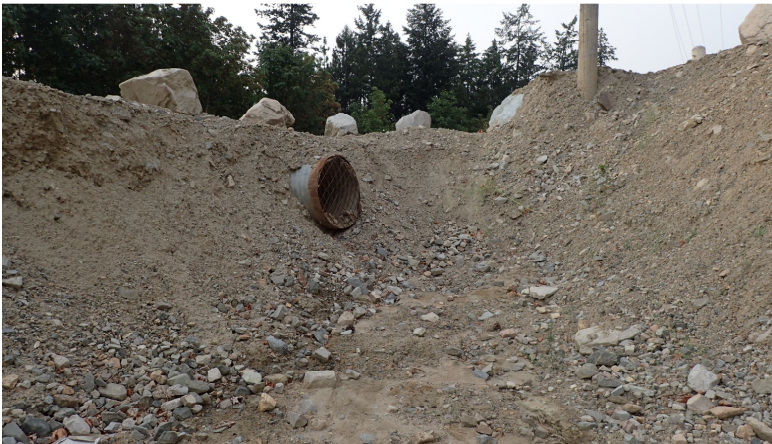
2018 August, viewing south to the 48" overflow culvert at the south end of the debris basin.
