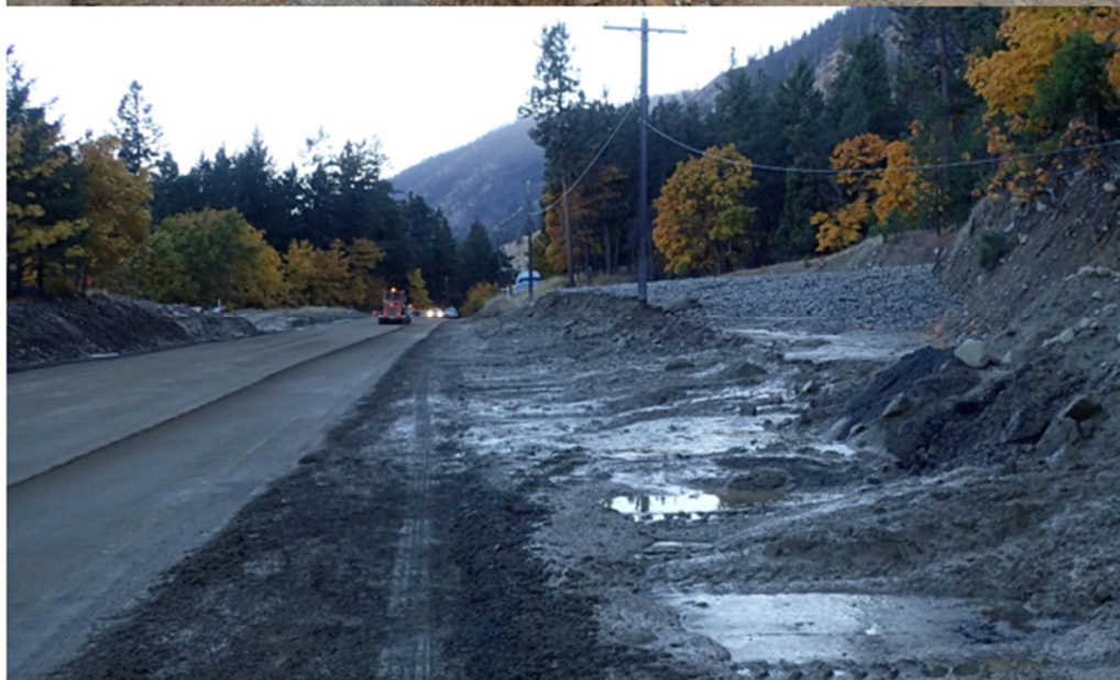
October 2017 event during emergency cleanup of road, prior to re-opening.
