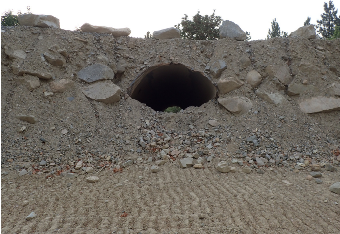
2018 August, looking at inlet of primary culvert from debris basin.
