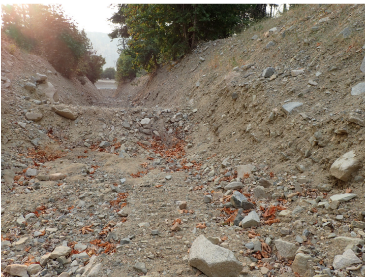
2018 August, viewing downstream at a check dam. Typical channel conditions for post-maintenance, prior to and debris deposition.
