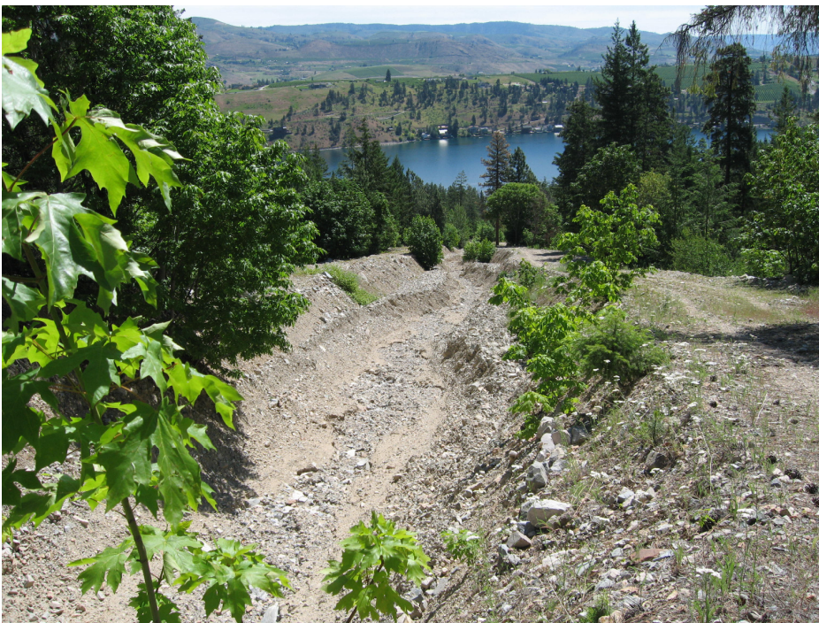
June 14, 2010 photo showing multiple debris flows with storage in upper channel. Taken about mid-way upstream from road to channel bend.
