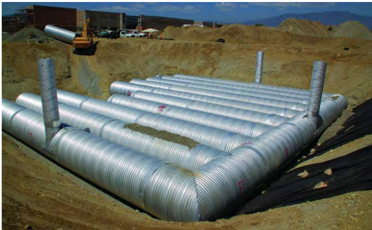
Figure 40. Example of a CMP stormwater gallery. Copied from Contech Engineered Solutions.
