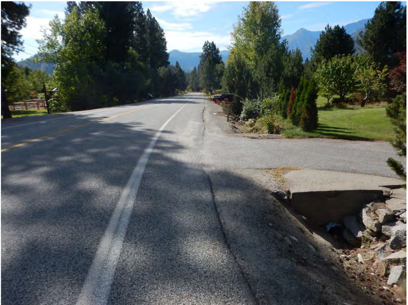
Figure 16. Partially blocked culvert along N-S Titus Road. The photo is taken from Point 6 on Figure 8.
