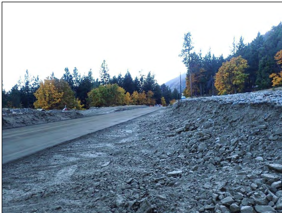
Figure 6: Deposited Debris in Sediment Basin after October 2017 Event, Looking South from Mouth of Drainage Channel
