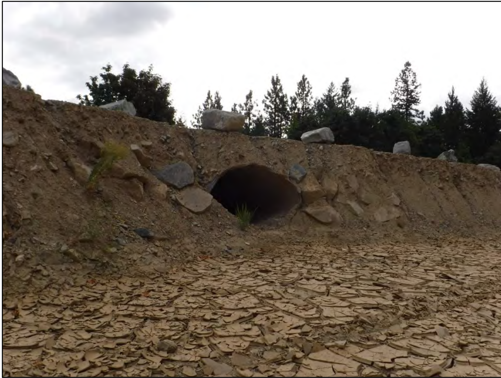
Figure 4: 96-Inch Culvert from the West Side of South Lakeshore Road
