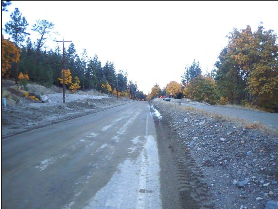
Figure 7: Sediment Basin to Left (West), Bypass Road to Right (East), Looking North after Debris Cleared from Roadway
