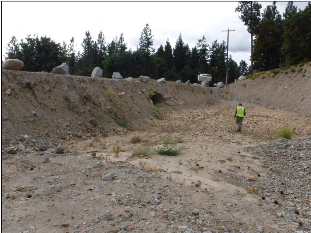
Figure 3: Sediment Basin Looking South From Mouth of Channel
