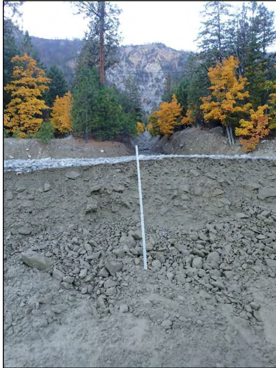
Figure 5: Deposited Debris in Drainage Channel after October 2017 Event (Looking West)
