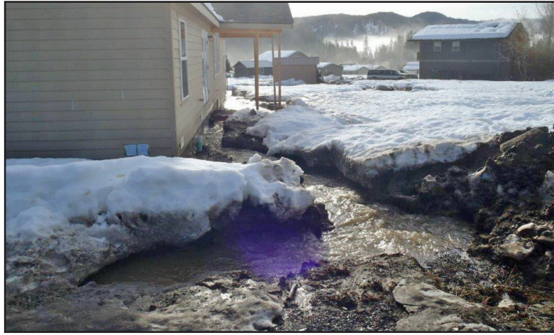
Ski Hill Basin 2016 spring runoff damages.
