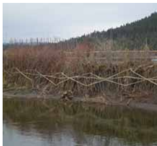
Stream bank stabilization with staking willow cuttings.
