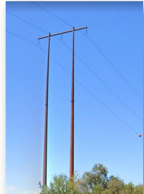
Typical 2-pole Structure 115KV Transmission
