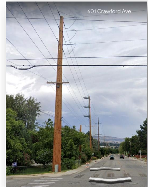
Typical 1-pole Structure 115KV Transmission
