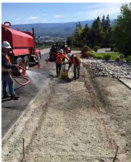
(Source: Chelan County Public Works)
