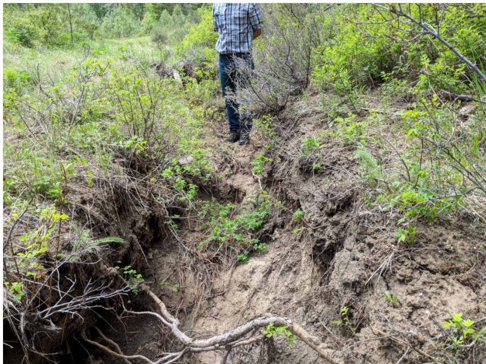
Figure 6. Showing severe erosion in the western Ns stream channels, where mitigation is proposed.
