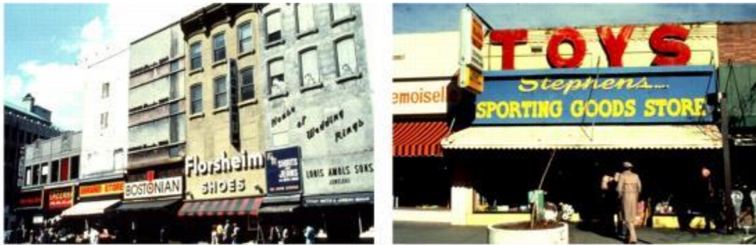
Figure 7. Unacceptable wall sign examples. These signs are out of scale with the facades and appear to cover over historical architectural features.
