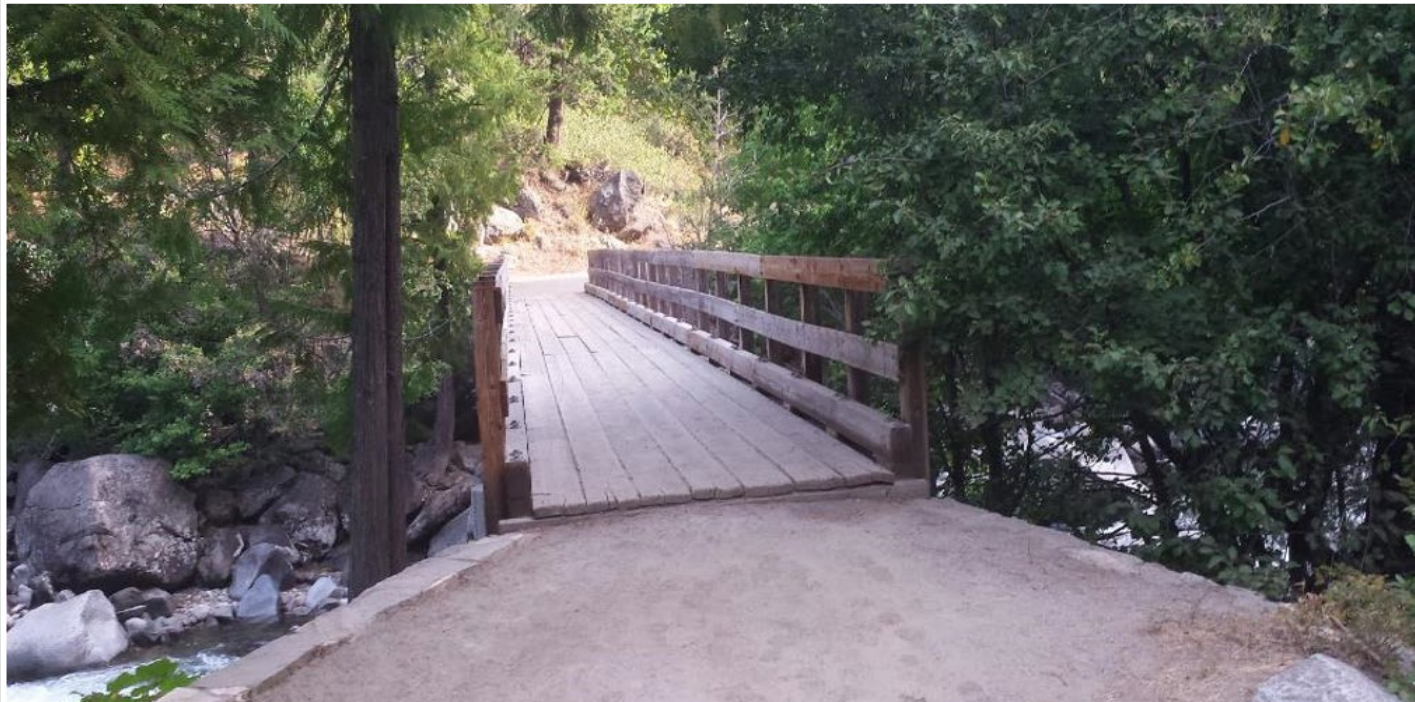
Snow Creek bridge
