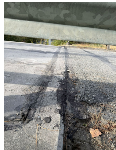
Peshastin Creek Bridge
