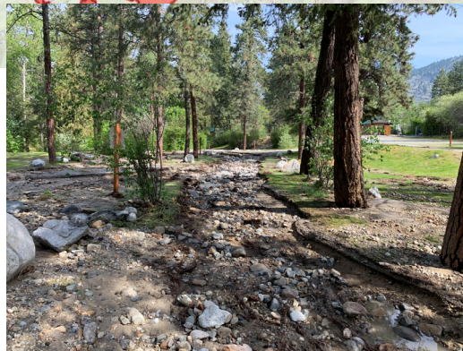
State Park Flood Damage
