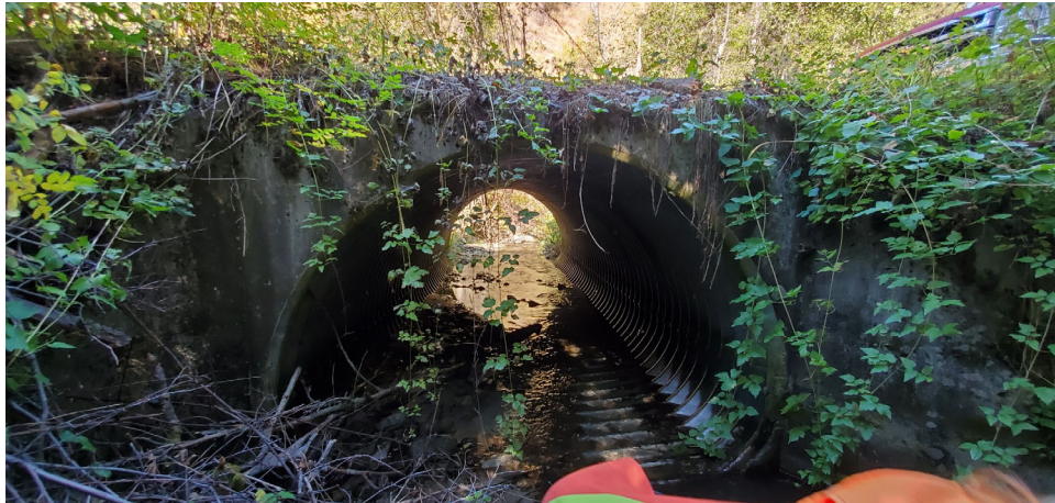
Sand Creek #3 Bridge Before Construction
