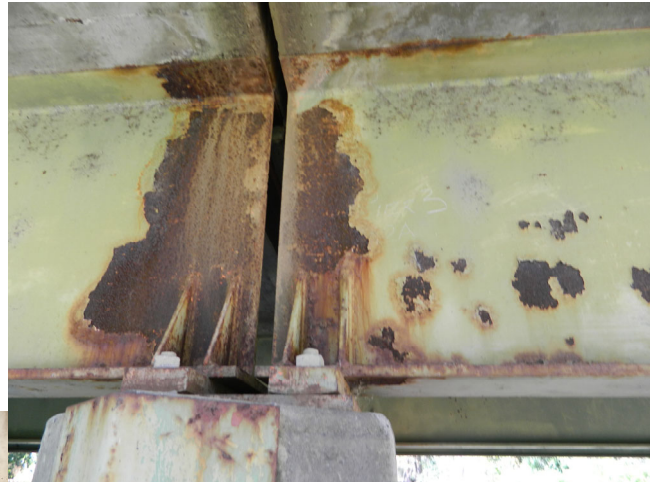
Painting Program Ardenvoir Bridge
