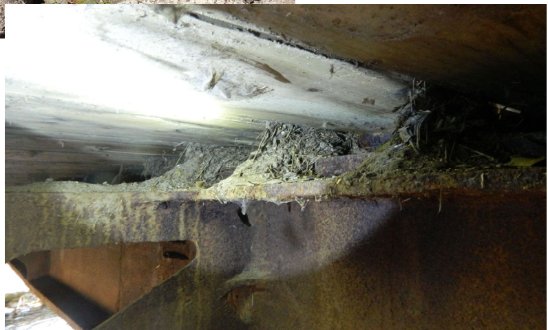
Bridge Cleaning Moe Ridge Bridge
