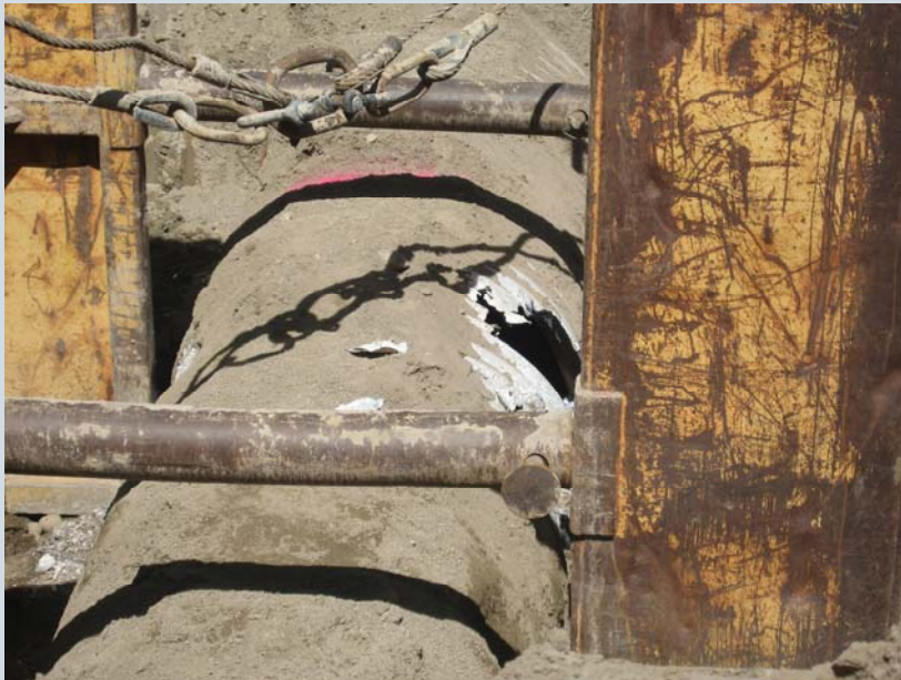
Picture shows deterioration of outfall pipe
