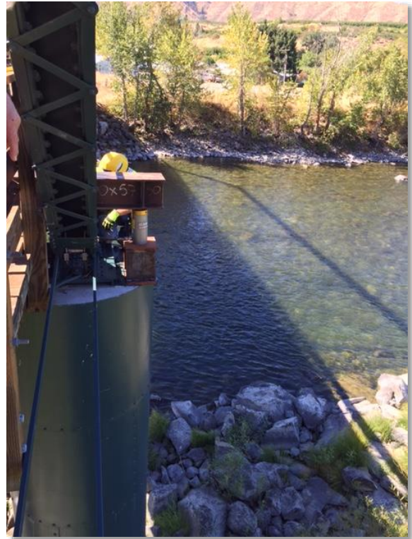
(Source: Chelan County Public Works)
