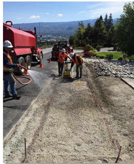
(Source: Chelan County Public Works)
