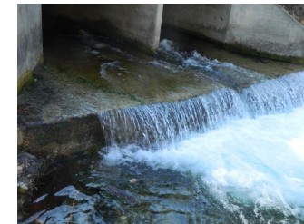
(Left) 25 Mile Creek Culvert
