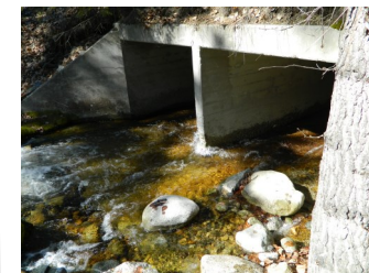
(Left) 25 Mile Creek Culvert
