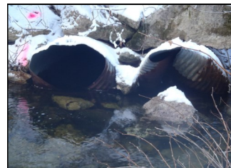
(Above) Washout of culverts from 2015 flood event.
