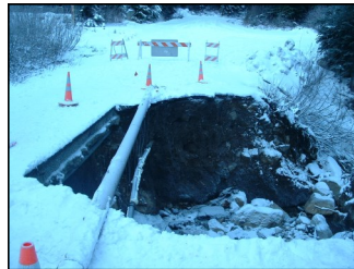
(Above) Washout of culverts from 2015 flood event.
