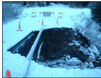
(Above) Washout of culverts from 2015 flood event.
