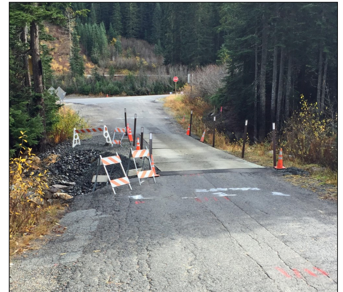
(Right) Temporary repairs to crossing included the installation of two culverts and road repairs.
