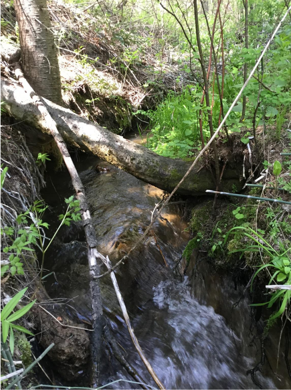
Bedrock in channel near proposed structure 10.
