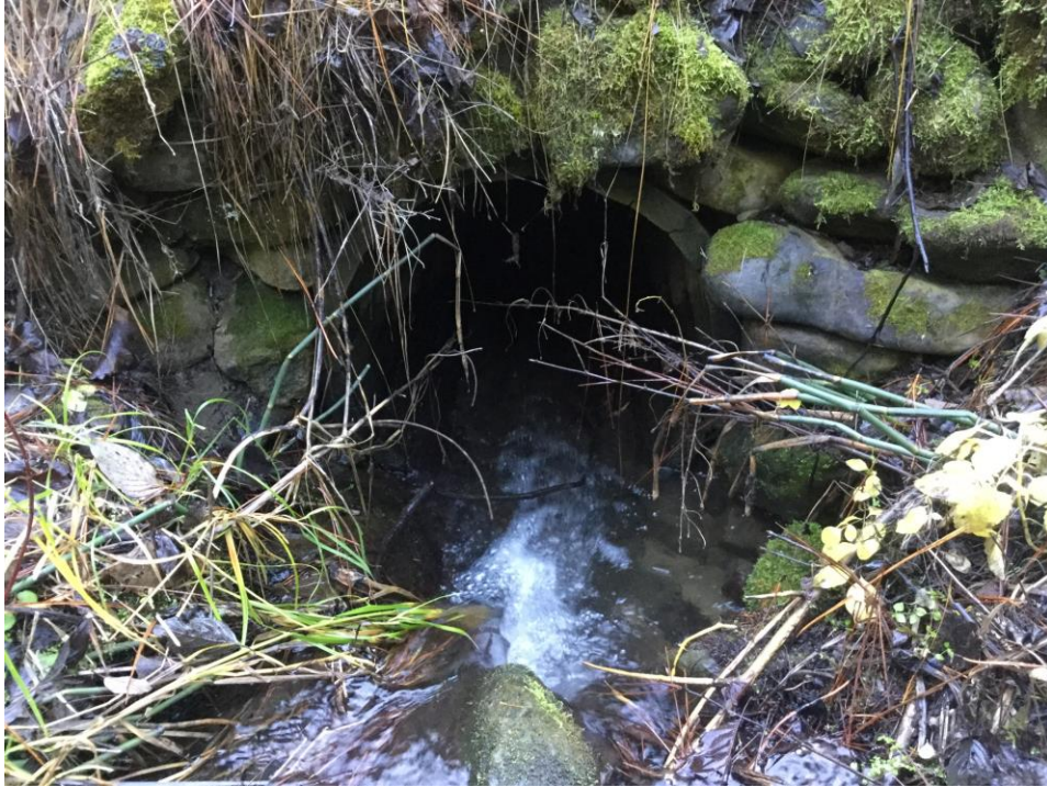
Figure 1. Poison Creek flowing through wooden culvert under FS Road 7104, just upstream of the confluence with Sand Creek (i.e., near RM 0.0). Photograph taken on 9 November 2016.
