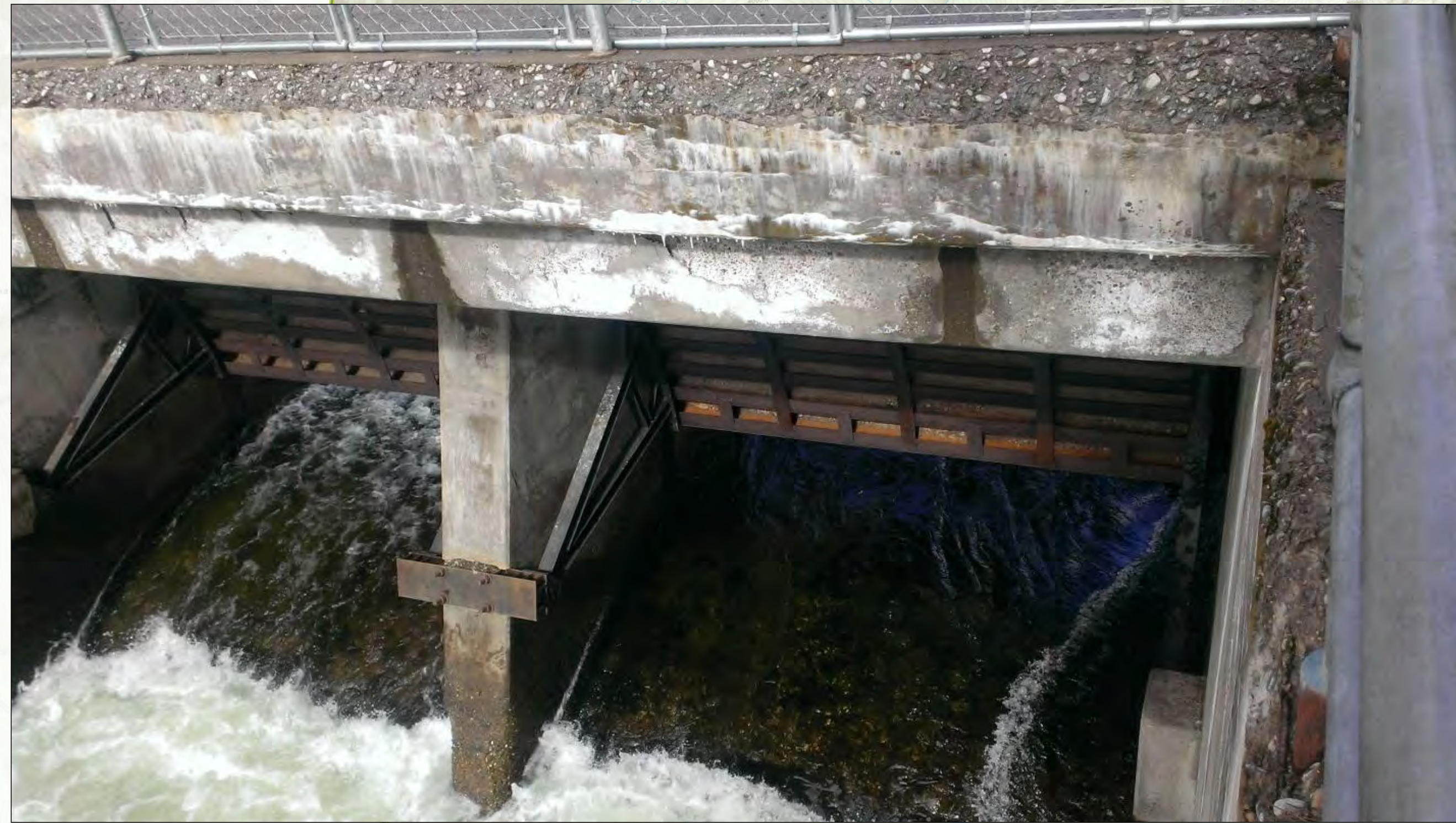
Radial Gate at Structure 2
