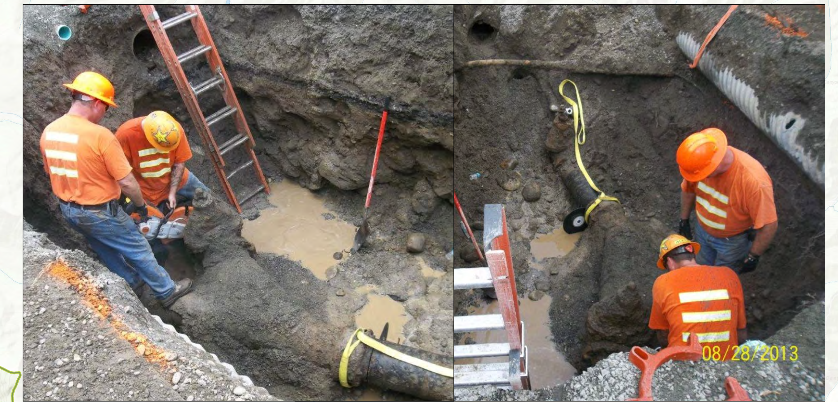
City of Leavenworth Pipe Rehabilitation
