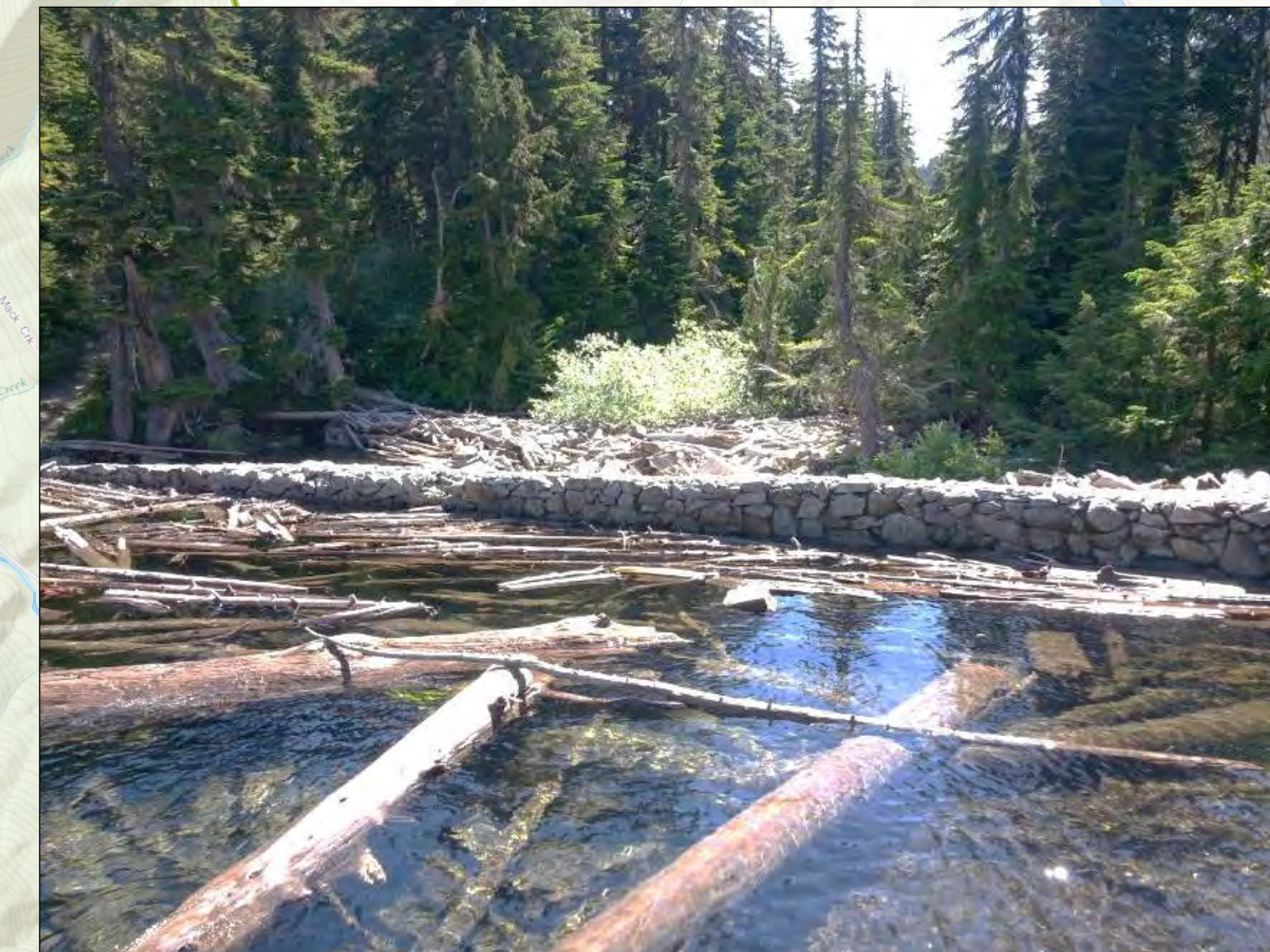
Square Lake Dam and Spillway
