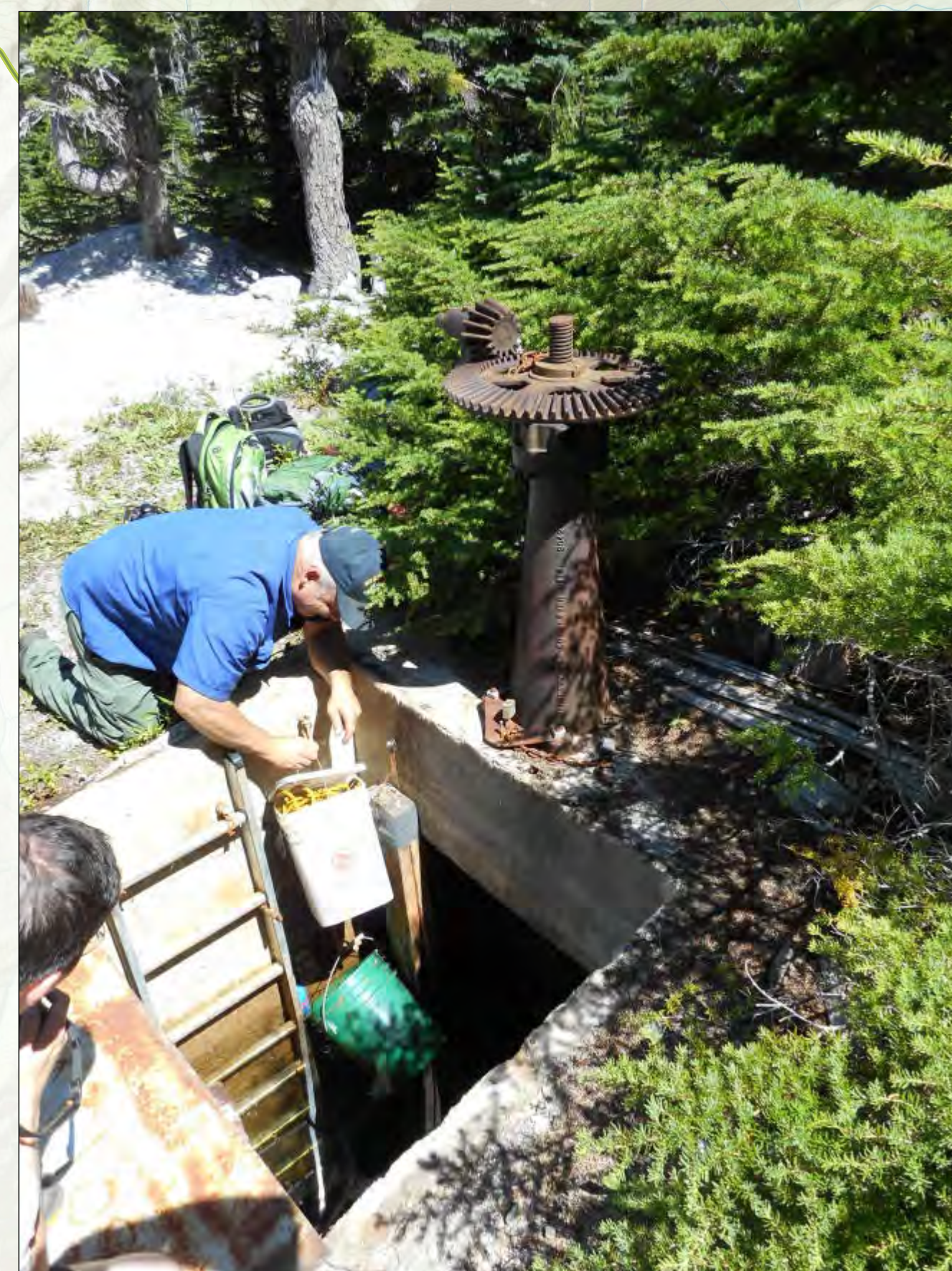
Lower Klonauqua Lake Gate Chamber Open with Gate Actuator
