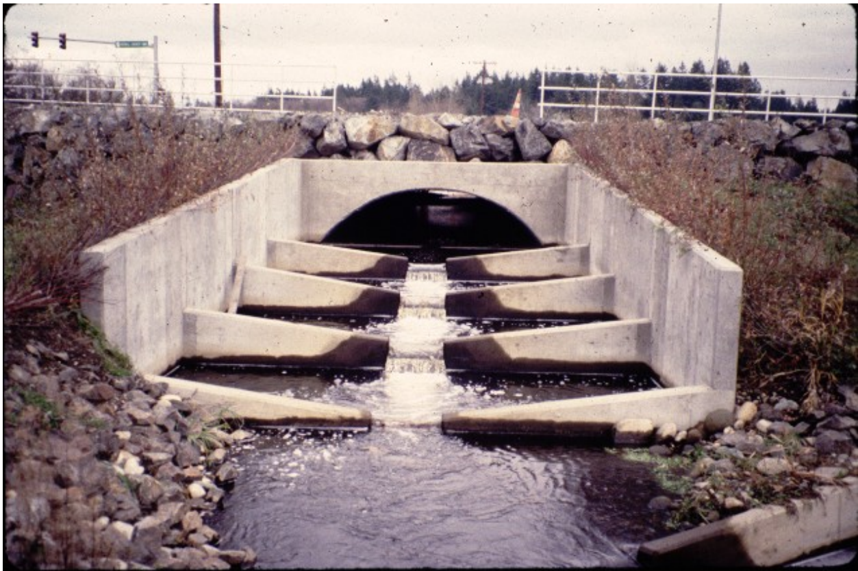
Photo 12 – Pool and Chute Fishway at low flow (Silver Creek, Washington).
