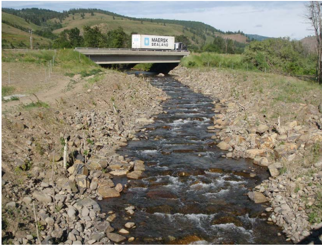
Photo 10 – Example of roughened channel fishway
