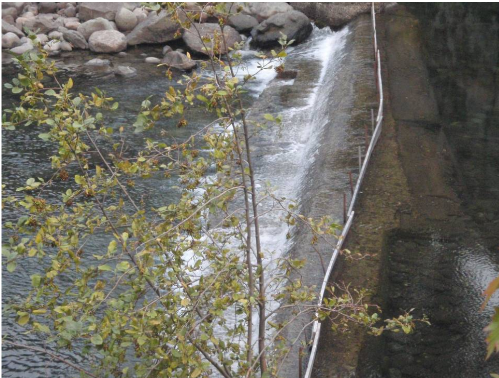
Photo 4 – Concrete Diversion Dam with flashboards at 20 cfs.
