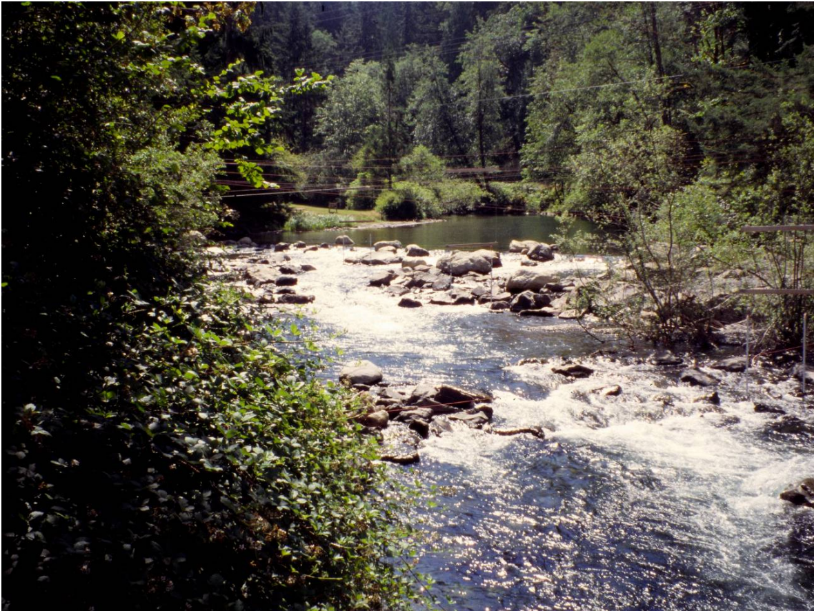
Photo 13 – Cedar River Constructed Riffle backwatering a 6-ft high concrete diversion dam
