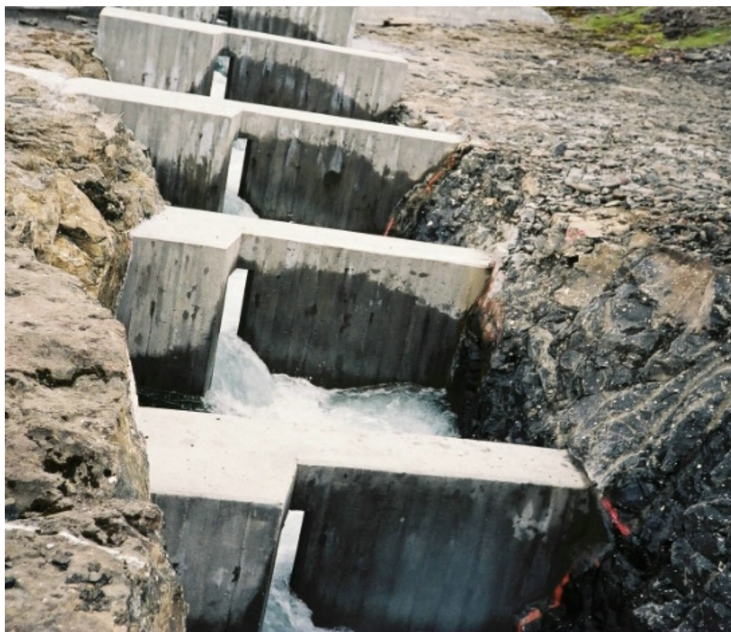
Photo 11 – Example of vertical slot fishway constructed within a rock trench excavated by blasting.
