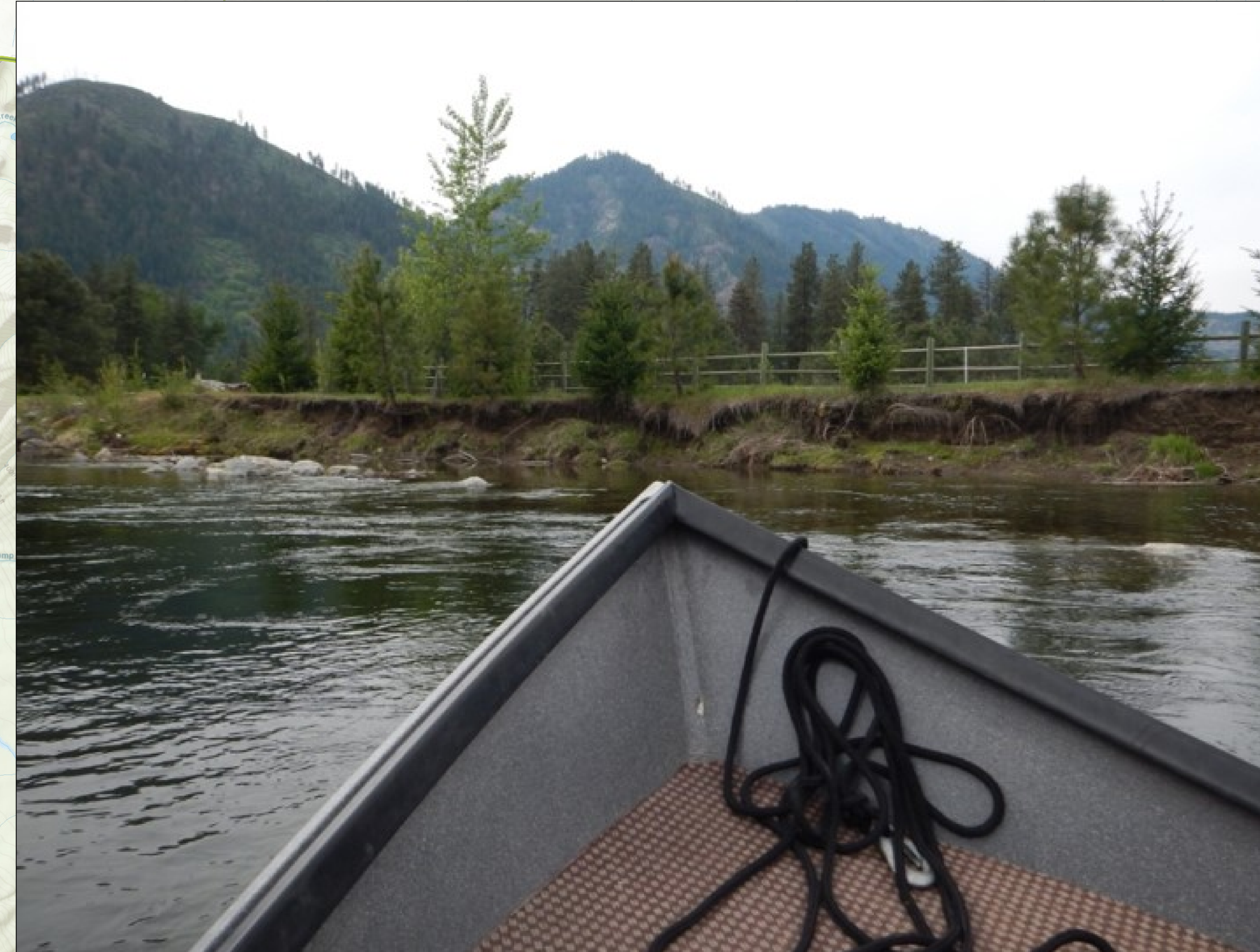
Eroding Banks, Icicle Creek
