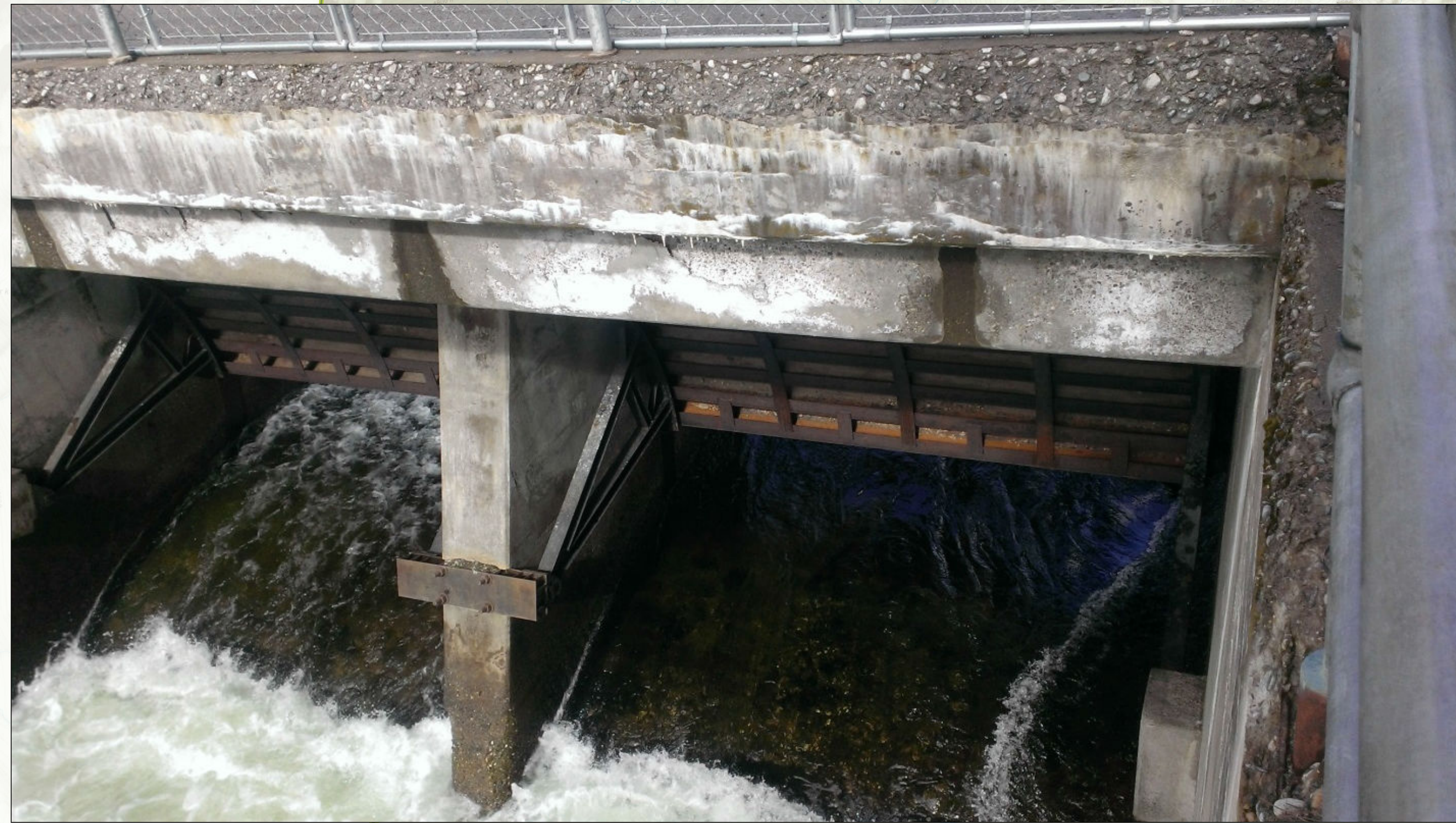
Radial Gate at Structure 2
