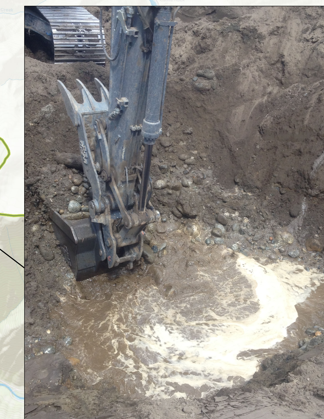
Groundwater Augmentation (Test Pits for proposed groundwater infiltration gallery on Hatchery Island)
