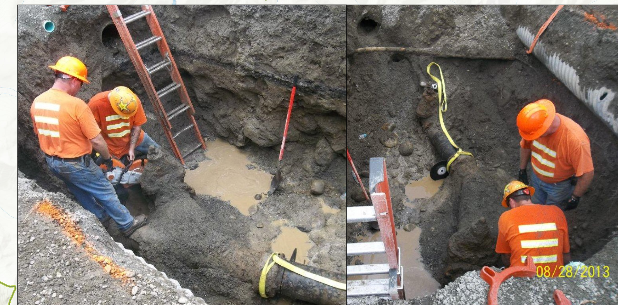
City of Leavenworth Pipe Rehabilitation
