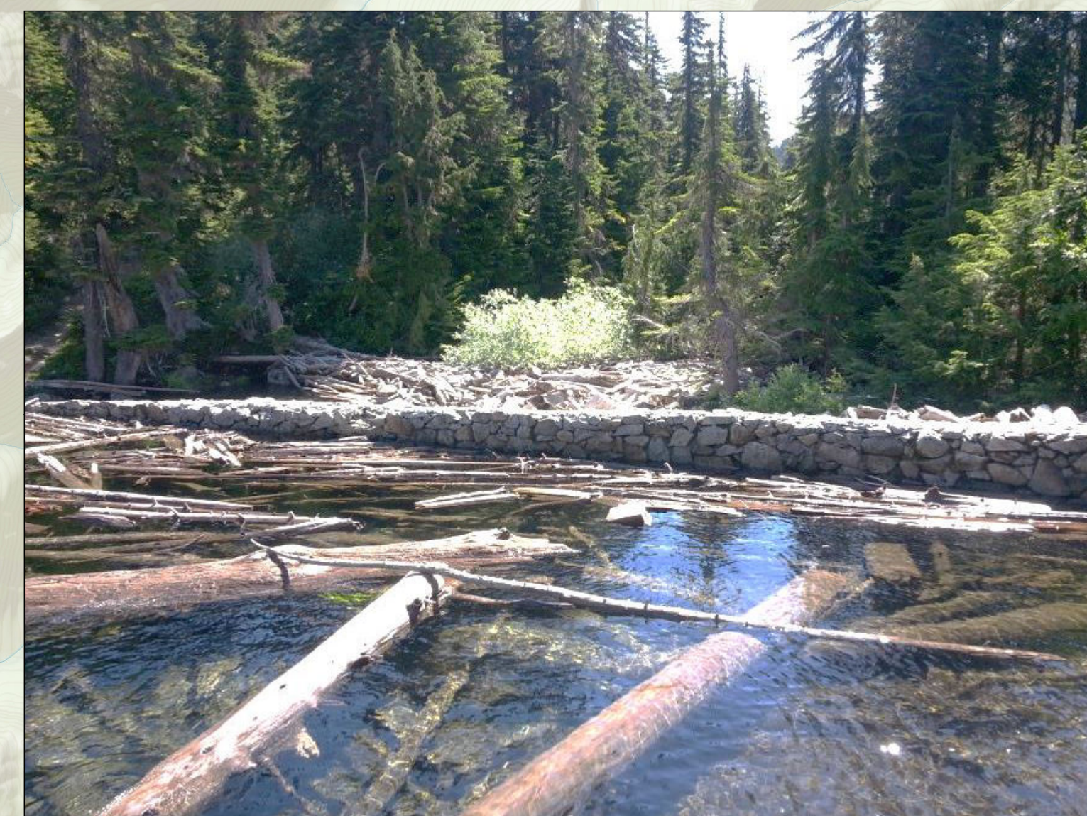
Square Lake Dam and Spillway
