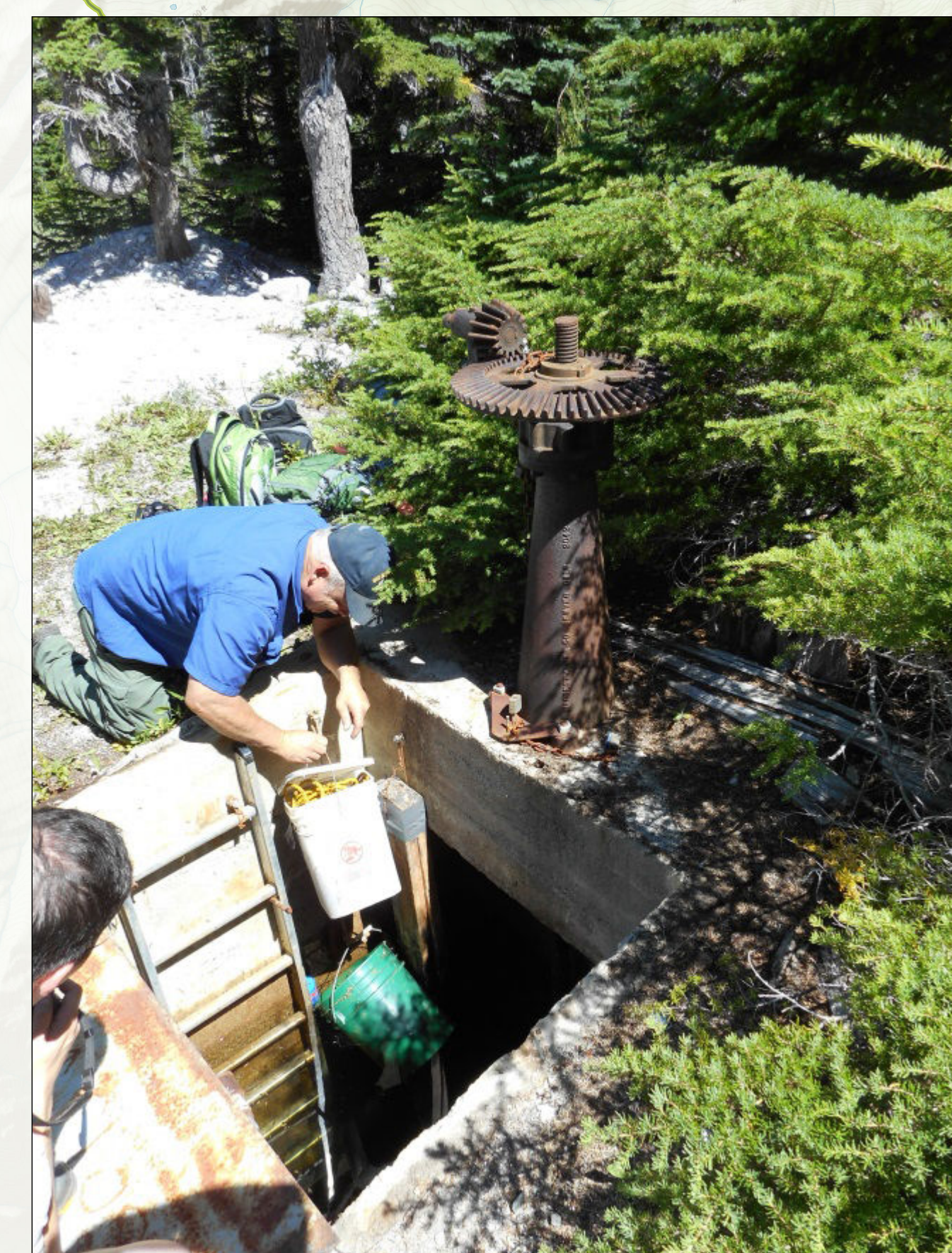
Lower Klonauqua Lake Gate Chamber Open with Gate Actuator
