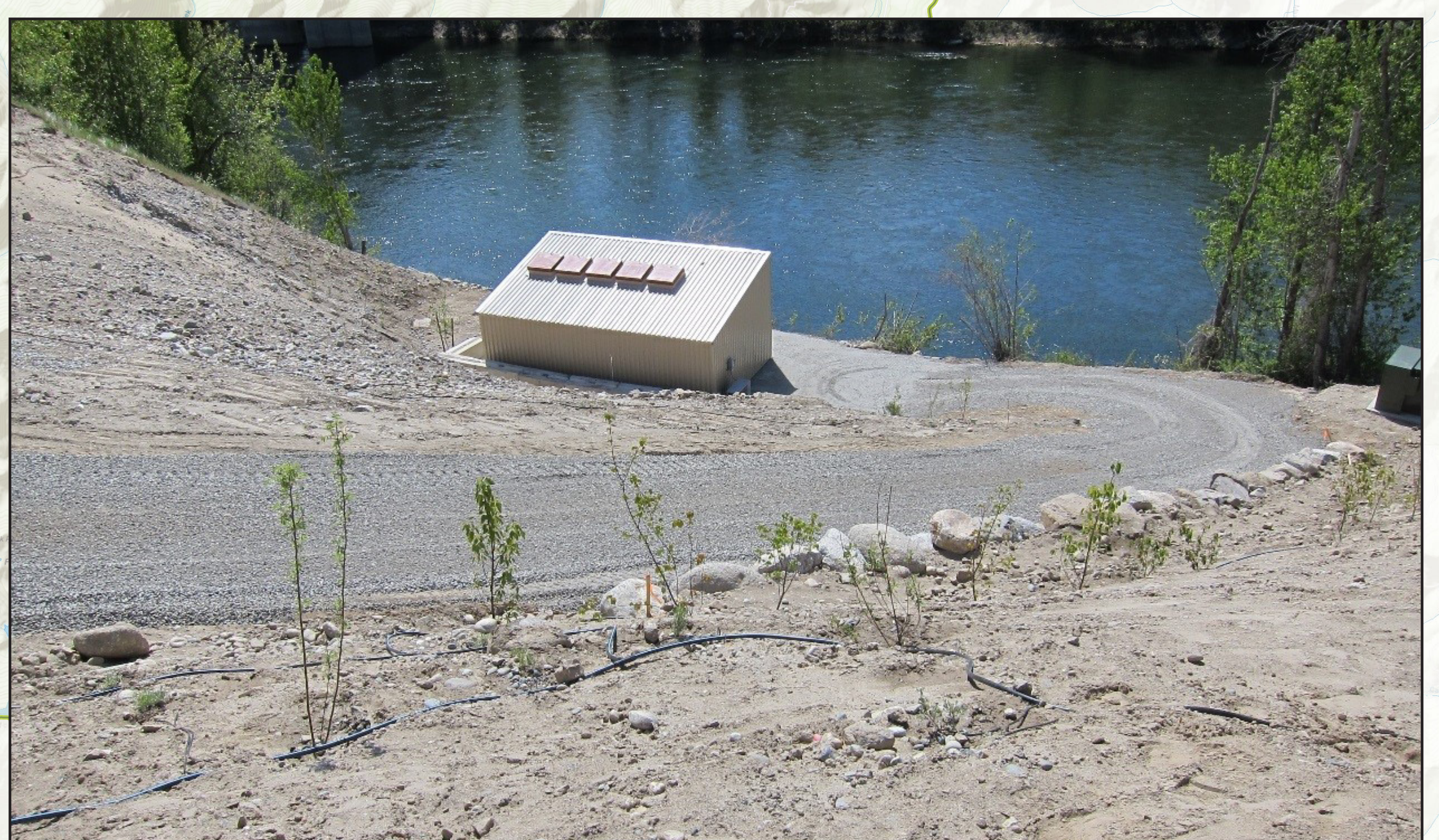
Example Pump Station Building
