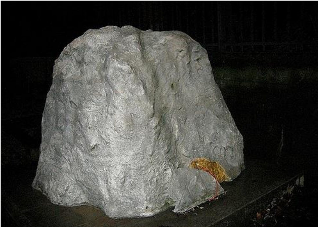
Figure 4-28. Representative Photo: Utility Cover
