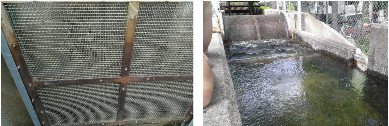
Figure 2-51. LNFH/COIC Fixed Plate Screen (left) and COIC Bypass Screen (right)
