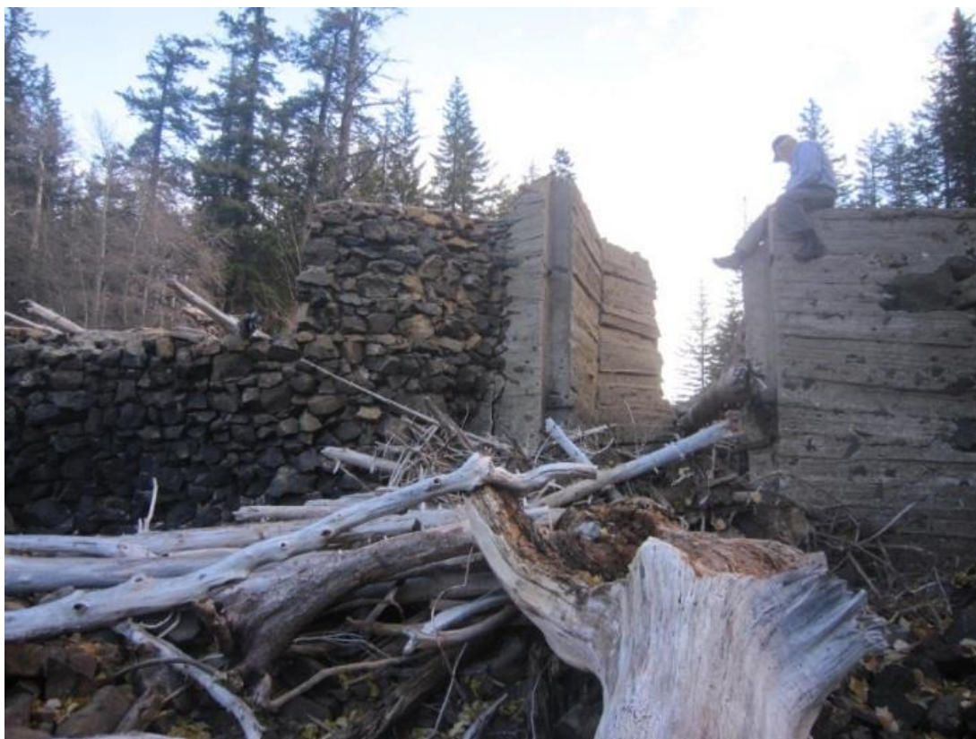
Figure 2-28. Current Alpine Lakes Infrastructure, Eightmile Dam (2015)
