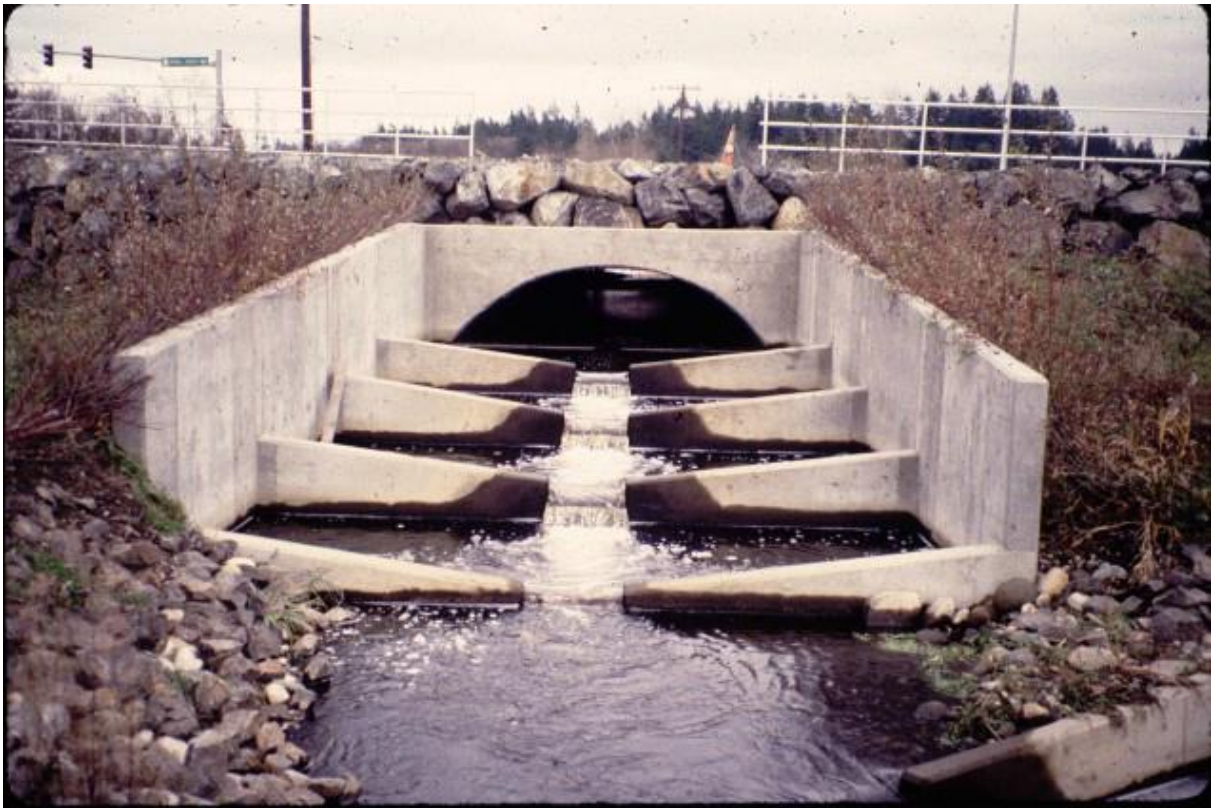
Figure 2-50. Example of pool and chute fishway
