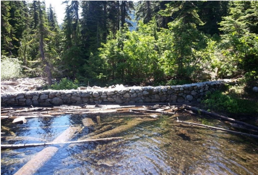
Figure 2–32. Current Alpine Lakes Infrastructure, Square Lake Dam
