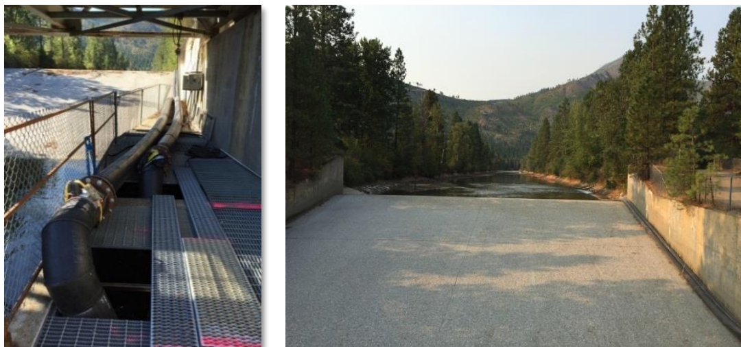
Figure 2-46. Effluent Pump Back Pilot Program
