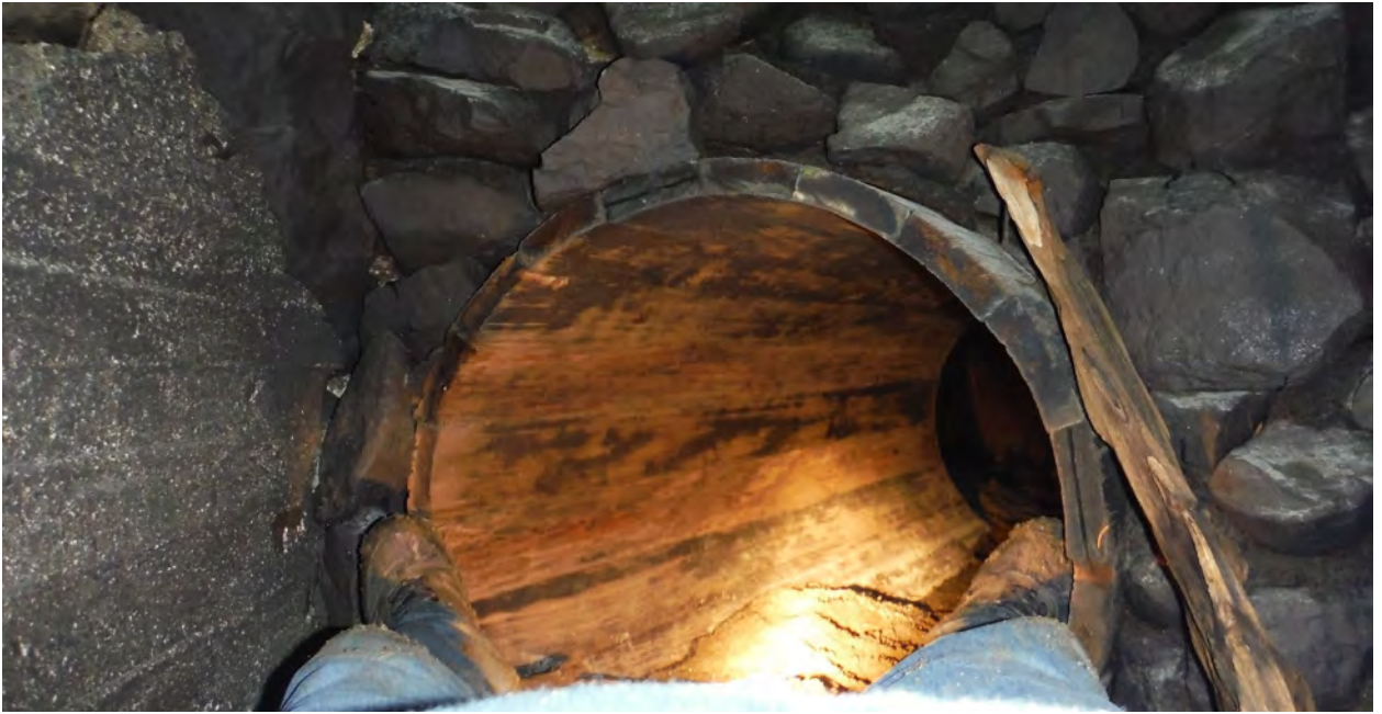
Photograph 10 Low-Level Outlet Pipe, Wood-Stave Section
