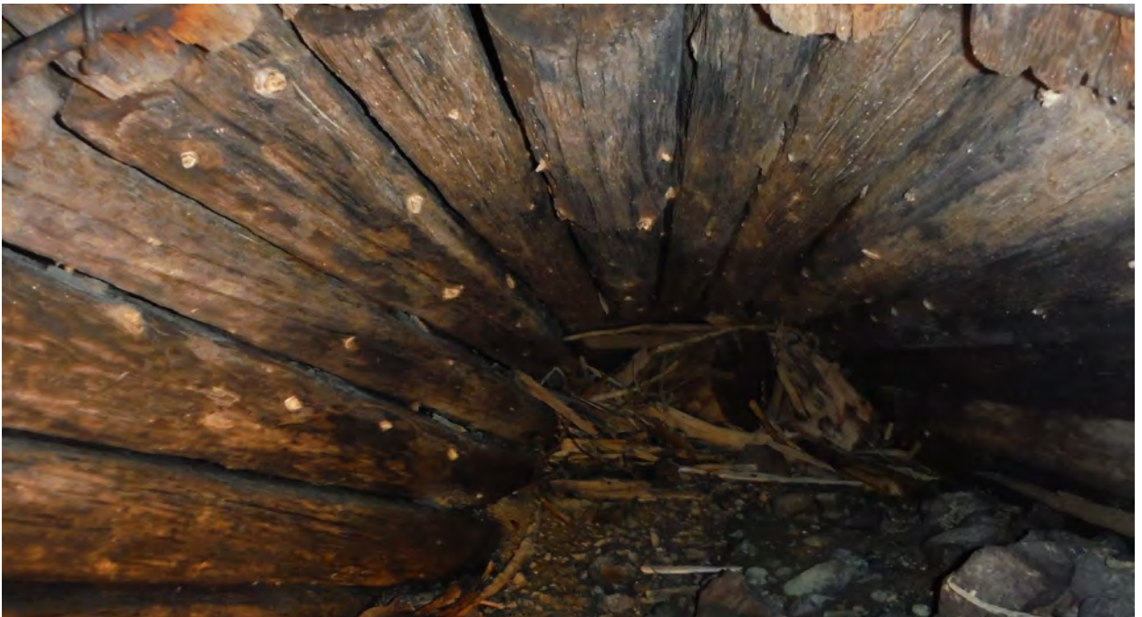
Photograph 9 Low-Level Outlet Pipe, Log-Stave Section
